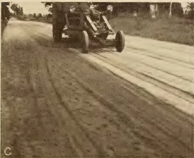
FIGURE 5.—STEPS IN SOIL ROAD CONSTRUCTION IN MICHIGAN. A, SCARIFYING OLD SURFACE; B, REMOVING LARGE STONE WITH RAKE; C, SPREADING PULVERIZED CLAY ADMIXTURE; D, DEEP BLADING TO MIX CLAY WITH OLD ROAD MATERIAL; E, SPREADING CHEMICAL OVER SMOOTHED SURFACE; F, MIXING BY BLADING IN WINDROWS.
