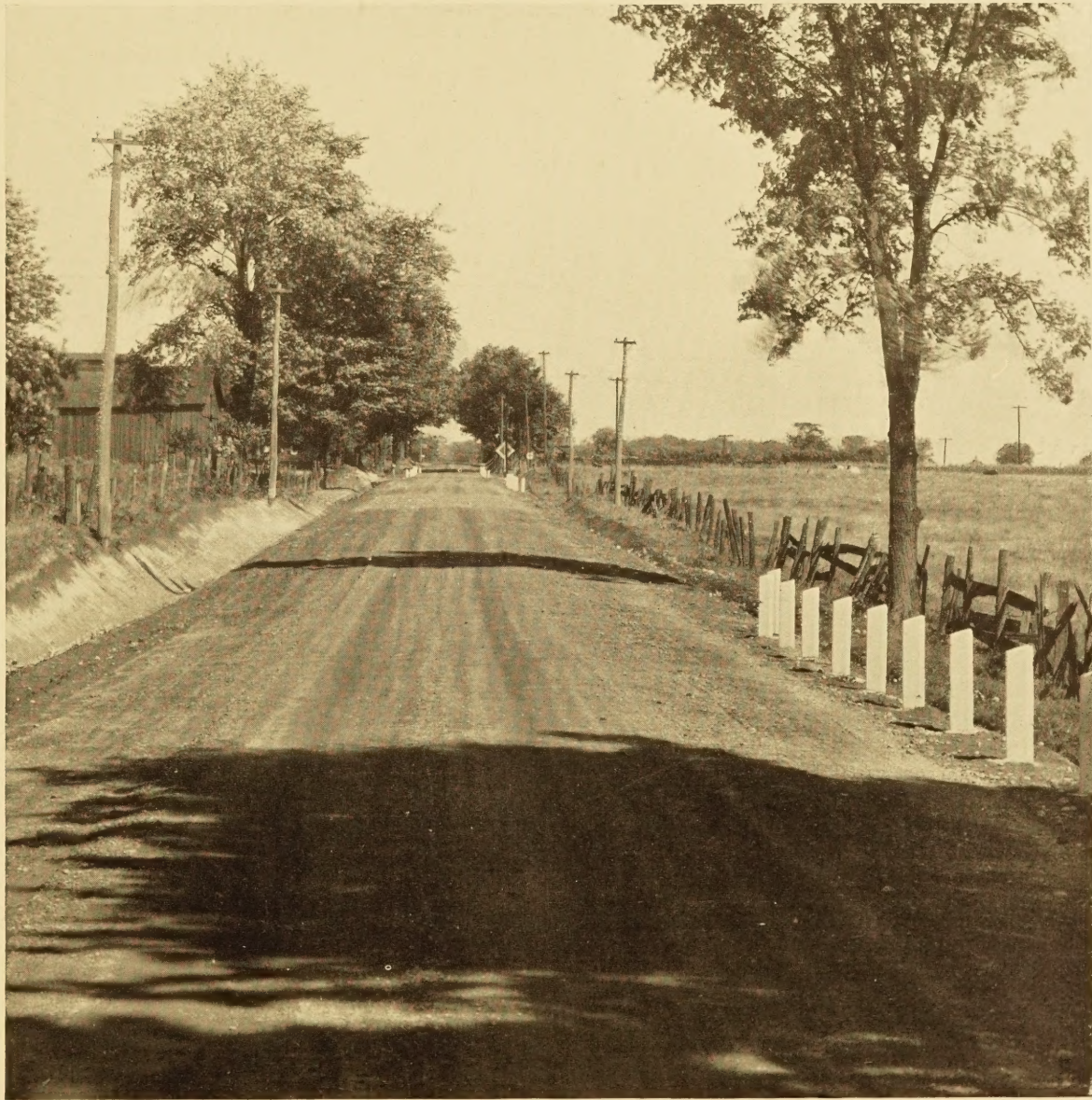
A SOIL ROAD IN ONONDAGA COUNTY, NEW YORK
