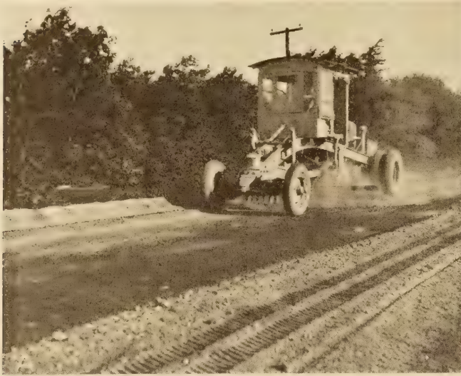
FIGURE 6.—A, SPREADING DRY MATERIAL OVER WETTED ROAD BED; B, ROLLING THE PARTIALLY DRY SURFACE.
