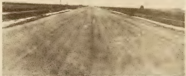
FIGURE 14.—A TYPICAL MINNESOTA GUMBO ROAD IN EARLY SPRING AND A ROAD ON SAME TYPE OF SOIL AFTER BEING TREATED WITH BITUMINOUS MATERIAL AND COVERED WITH A THIN LAYER OF GRAVEL.
