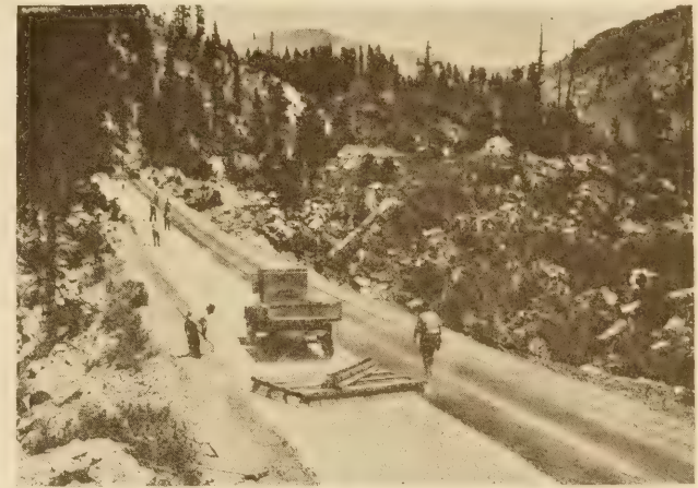
FIGURE 7.—TOUCHING UP SURFACE BY HAND AND DRAGGING WITH A BROOM.
