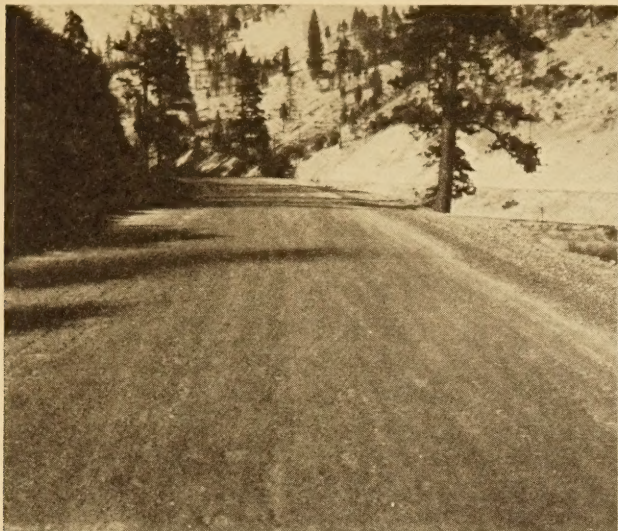
FIGURE 1.—TYPICAL CONDITION OF THE OLD SURFACE AT TIME OF CONSTRUCTION.
