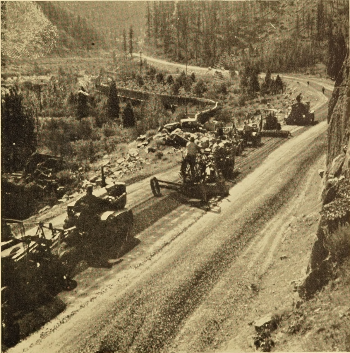
ROAD-MIX CONSTRUCTION IN CALIFORNIA
