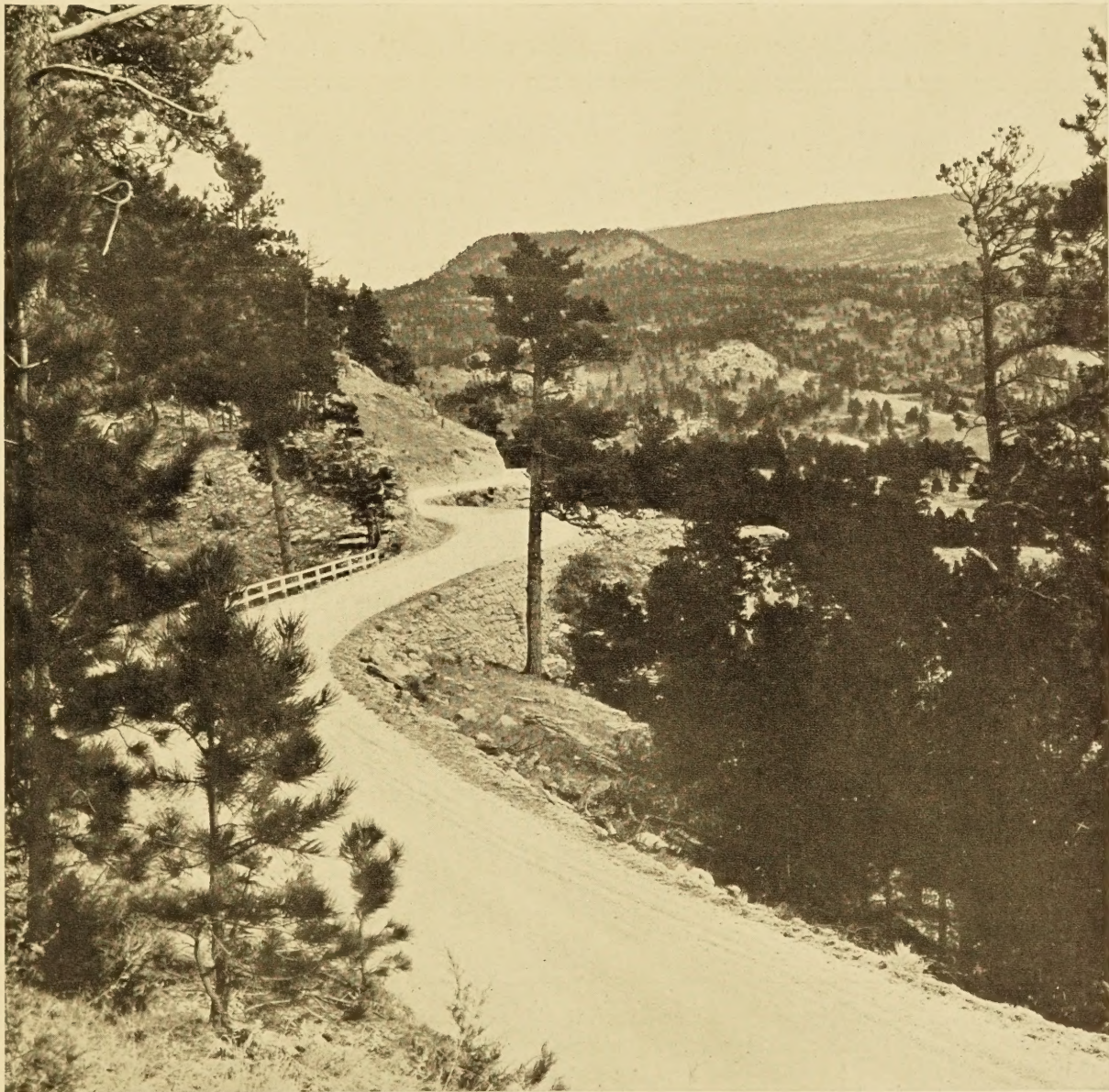
A SECTION OF U. S. 85 IN WYOMING
