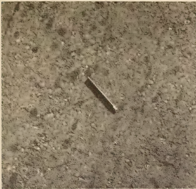
TYPICAL OIL-MIX SURFACES WHICH HAVE GIVEN EXCELLENT SERVICE. THE MIX SHOWN ON THE LEFT WAS RICH AND UNSTABLE THE FIRST YEAR AND WAS REMIXED WITH ADDITIONAL GRAVEL. IT WAS THREE YEARS OLD AT THE TIME OF INSPECTION. THE ONE ON THE RIGHT HAD RECEIVED NO MAINTENANCE OF ANY KIND SINCE ITS CONSTRUCTION FOUR YEARS PRIOR TO THE INSPECTION.
