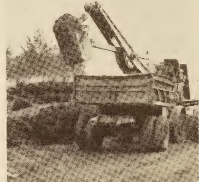
LARGE DIPPER LOADS ARE NECESSARY FOR HIGH PRODUCTION RATES.
