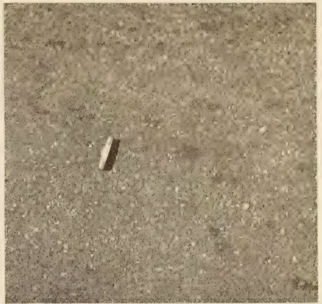
TYPICAL OIL-MIX SURFACES WHICH HAVE GIVEN EXCELLENT SERVICE. THE MIX SHOWN ON THE LEFT WAS RICH AND UNSTABLE THE FIRST YEAR AND WAS REMIXED WITH ADDITIONAL GRAVEL. IT WAS THREE YEARS OLD AT THE TIME OF INSPECTION. THE ONE ON THE RIGHT HAD RECEIVED NO MAINTENANCE OF ANY KIND SINCE ITS CONSTRUCTION FOUR YEARS PRIOR TO THE INSPECTION.
