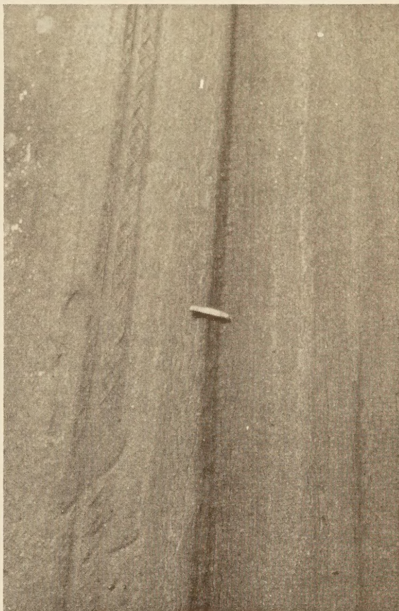
GENERAL VIEW AND DETAIL OF A SURFACE OF GROUP 1 WHICH WAS HIGHLY UNSTABLE DUE TO A HIGH COMBINED OIL AND WATER CONTENT. AGE APPROXIMATELY ONE YEAR AT TIME OF INSPECTION. NOTE TIRE MARKS AND FOOT TRACKS ON THIS SURFACE.
