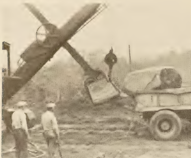
LARGE BOULDERS ARE HARD ON EQUIPMENT AND DECREASE THE RATE OF PRODUCTION. THEY SHOULD BE REDUCED BY BLASTING.
