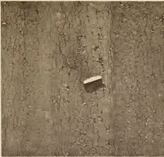
TYPICAL EXAMPLES OF FAILURE CAUSED BY HIGH MOISTURE CONTENTS IN THE MIXTURES. THESE GROUP 1 SURFACES ARE TWO AND THREE YEARS OLD.
