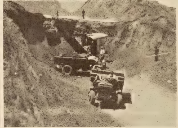
EXAMPLES OF CORRECT "SPOTTING" OF TRUCKS FOR LOADING WITH SHORT SWING OF SHOVEL.
