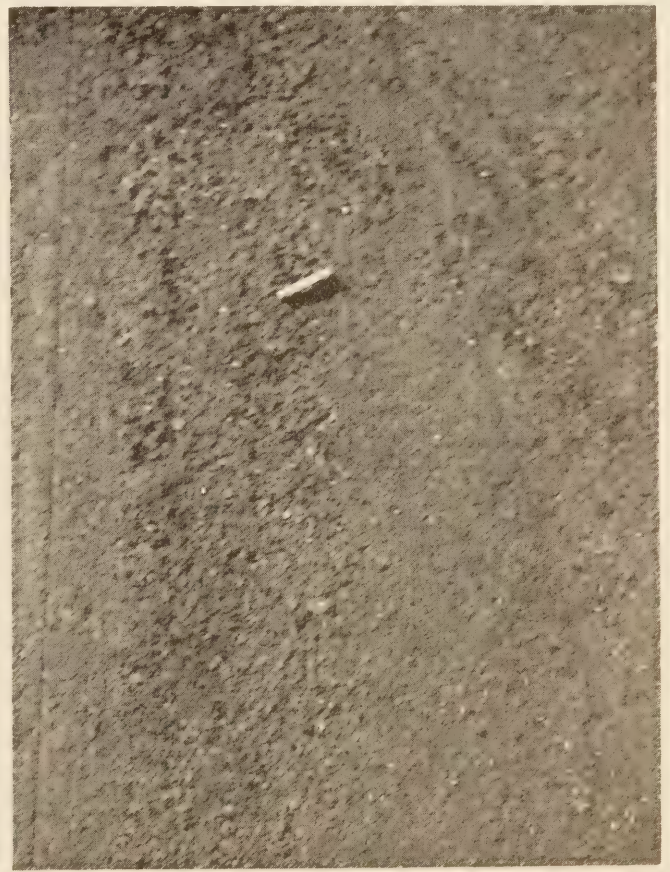
TYPICAL EXAMPLES OF RAVELING OF GROUP 3 SURFACES HAVING A LOW OIL CONTENT AND NO SEAL COAT OR SURFACE TREATMENT TO PREVENT LOSS OF AGGREGATE.
