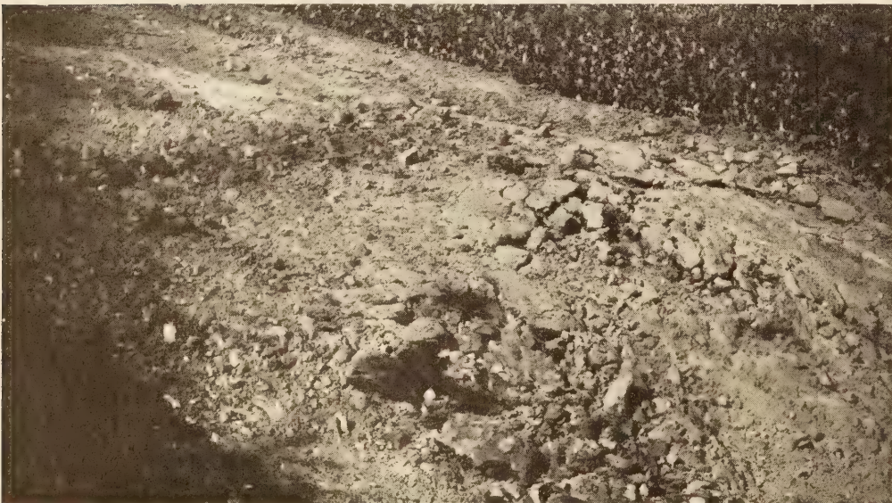
APPEARANCE OF GROUND AFTER A SATISFACTORY BLAST. MATERIAL WELL BROKEN BUT NOT SCATTERED.
