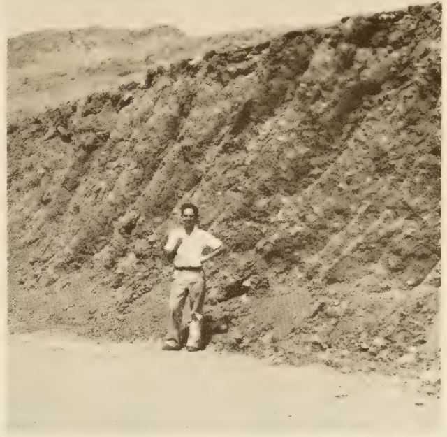
MATERIAL TOO HARD TO DIG READILY WITHOUT BLASTING.
