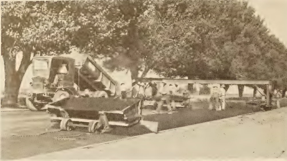
INITIAL SPREADING WITH SPREADER BOXES.
