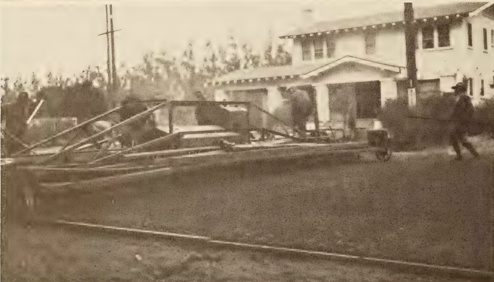
FINAL SPREADING WITH FINISHING MACHINE.
