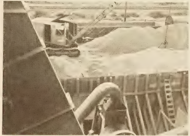
MATERIALS YARD, AND ARRANGEMENT OF BULKHEADS. DUST COLLECTOR IN FOREGROUND.
