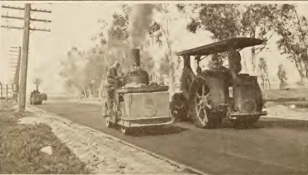
STEPS IN SPREADING AND ROLLING.
