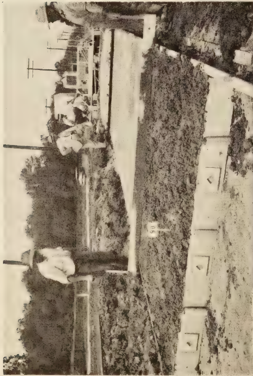
LEFT: ROUGHLY LEVELED CONCRETE READY TO BE STRUCK OFF.
