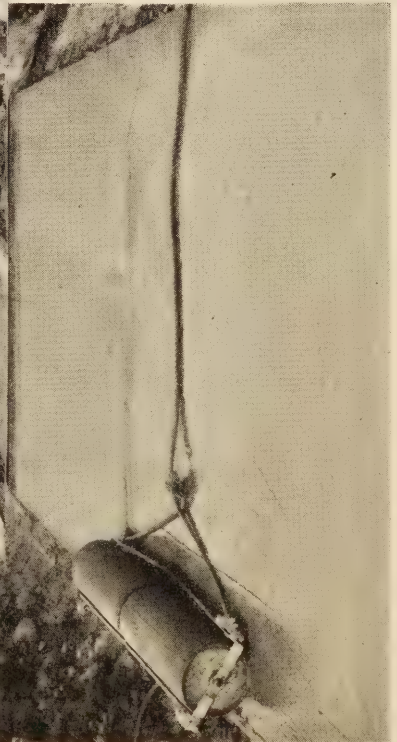
LEFT: ROLLING SURFACE WITH LIGHT SHEET- METAL ROLLER.
