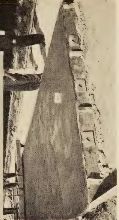
LEFT: ROLLING SURFACE WITH LIGHT SHEET- METAL ROLLER.
