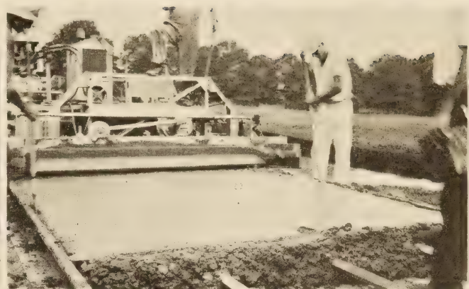
AFTER FIRST PASSAGE OF FINISHING MACHINE.
