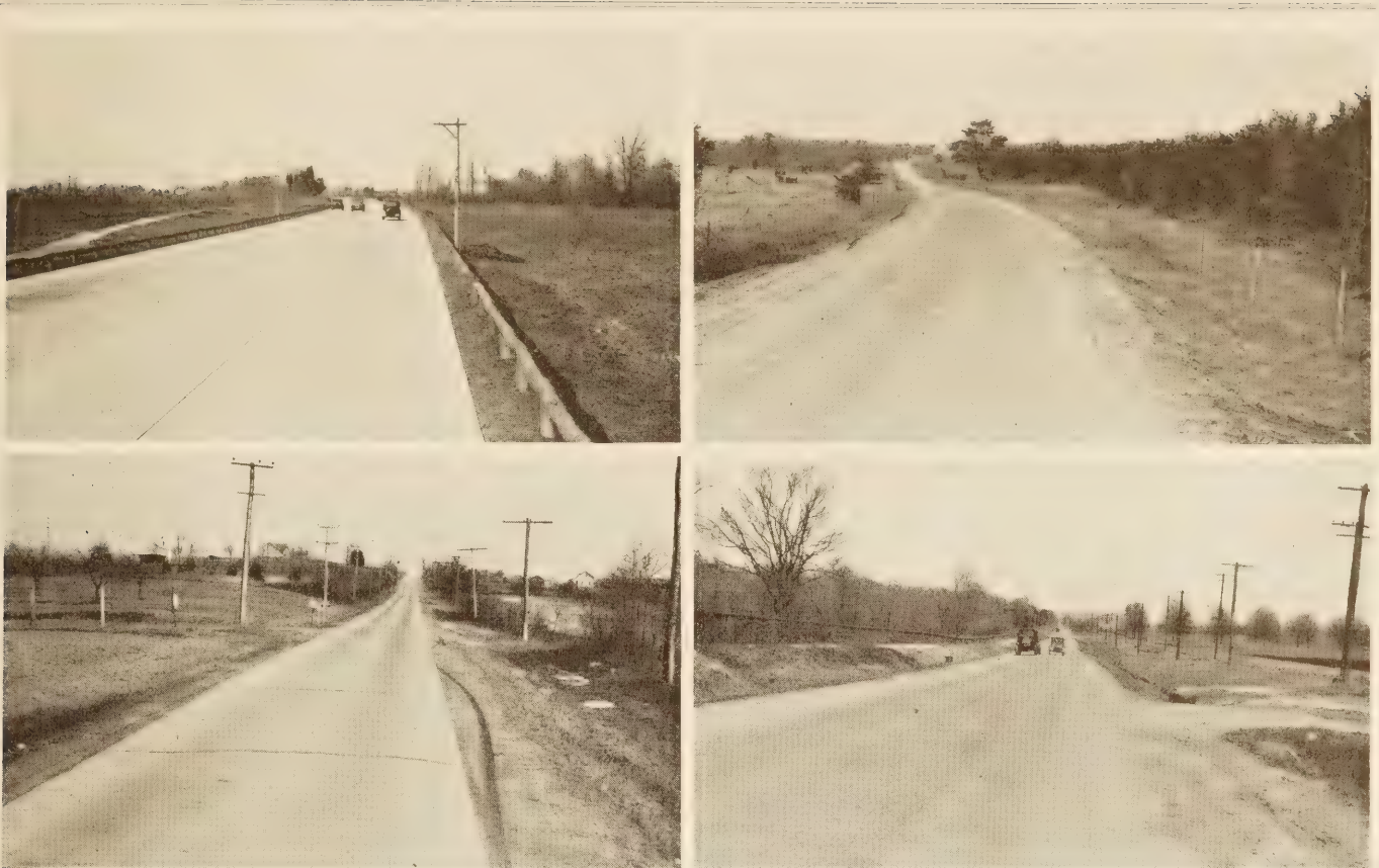
UPPER.—THE SMOOTHEST CONCRETE SURFACE TESTED LOWER.—THE ROUGHEST CONCRETE SURFACE TESTED
