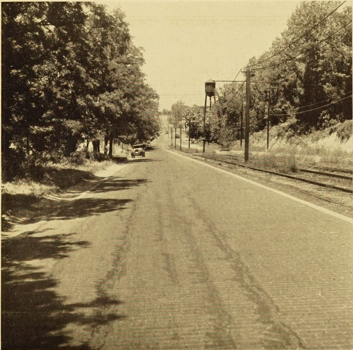
A BRICK PAVEMENT 19 YEARS AFTER ITS CONSTRUCTION
