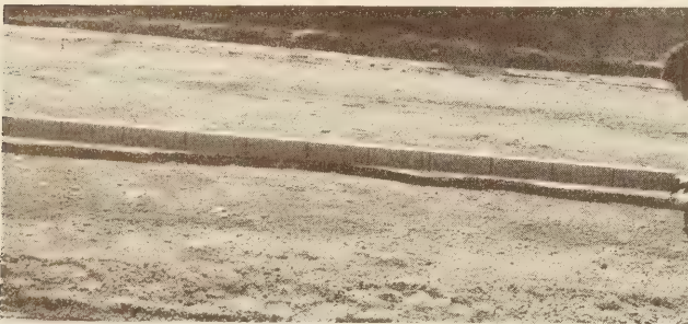
FIGURE 20.—IMPACT REACTIONS PRODUCED ON A CONCRETE ROAD AT A SHARP VERTICAL CURVE AT THE TOP OF A HILL
