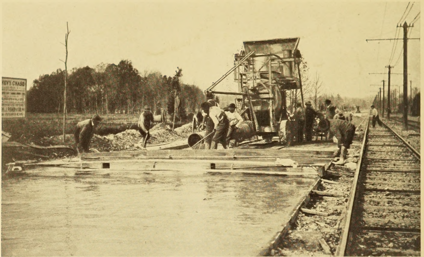
CONCRETE CONSTRUCTION ON CONNECTICUT AVENUE EXPERIMENTAL ROAD, NOVEMBER, 1912
