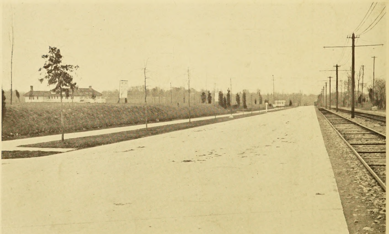
CONDITION OF CONCRETE SURFACE IN APRIL, 1914
