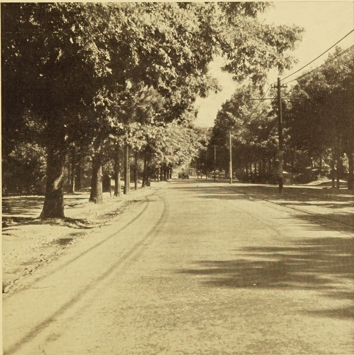
A BITUMINOUS MACADAM ROAD AFTER 21 YEARS OF SERVICE
