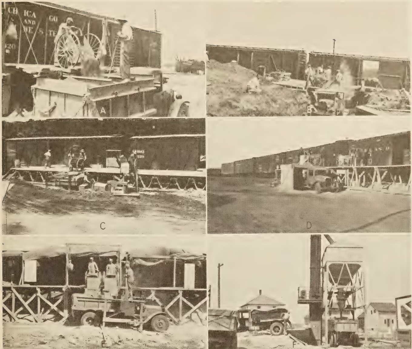
FIGURE 4.—HANDLING BULK CEMENT:
