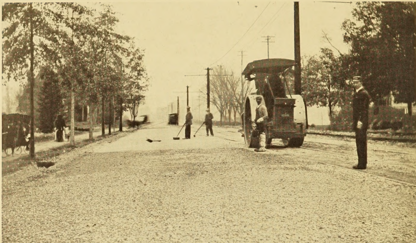
CONNECTICUT AVENUE EXPERIMENTAL ROAD, CHEVY CHASE, MD., NOVEMBER, 1911, SHOWING APPLICATION OF SEAL COAT IN THE FOREGROUND AND FINISHED BITUMINOUS MACADAM ROAD IN THE DISTANCE
