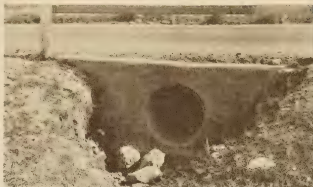
INLET END (WEST)
