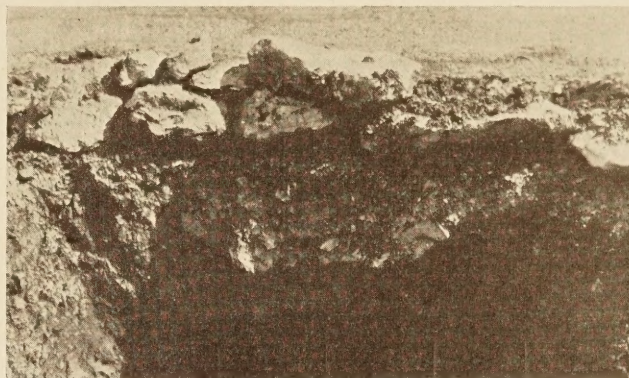
INLET END (WEST)
