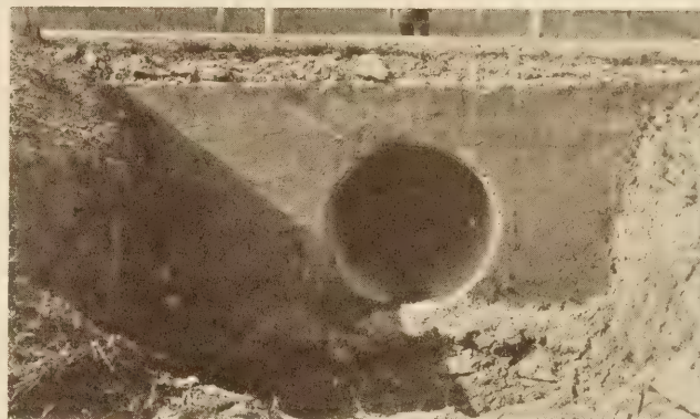
OUTLET END (EAST)
