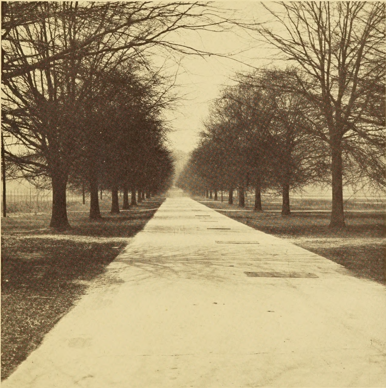
RUNWAY WITH ARTIFICIAL OBSTRUCTIONS USED IN IMPACT TESTS AT ARLINGTON
