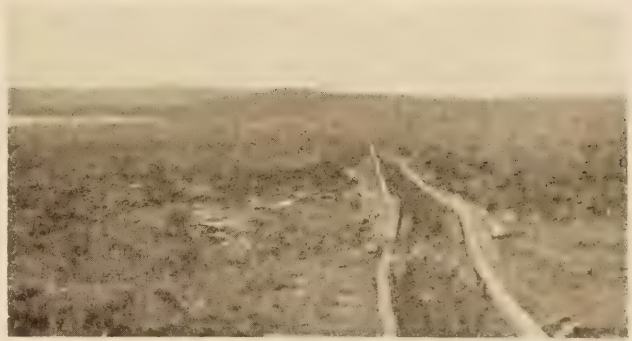
FIGURE 21.—EFFECT OF HEAVE AND THRUST ON THE POSITION OF A TRAM LINE IN ALASKA. (PHOTO BY U. S. G. S.)
