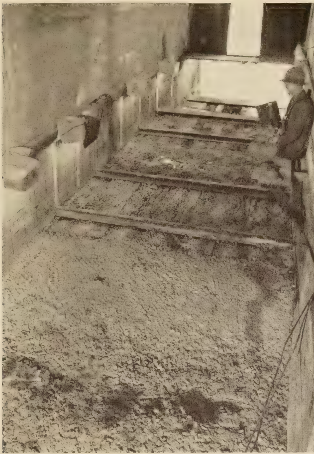
FIGURE 3.—DOUBLE-TRACK EMBANKMENT WITH RAILS IN PLACE
