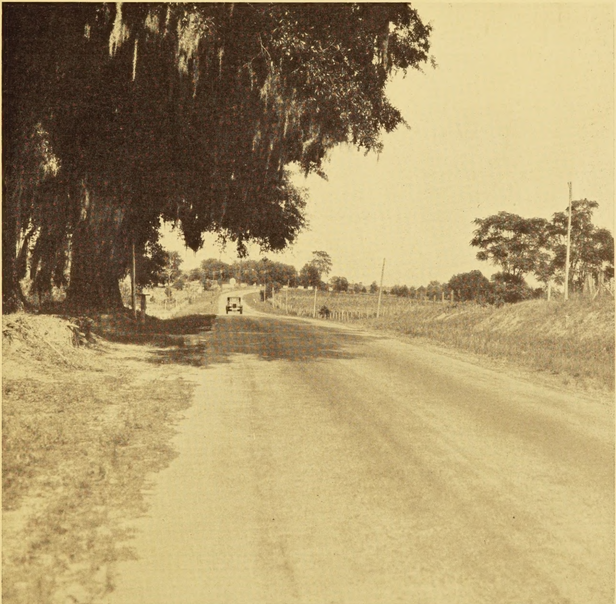
AN EXAMPLE OF THE SURFACE OBTAINED BY SURFACE TREATING SAND-CLAY AND TOPSOIL ROADS
