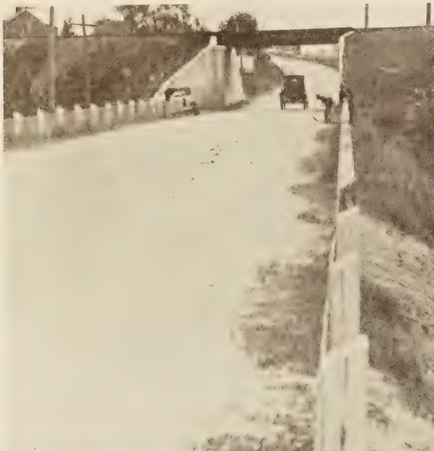
SURFACE TREATED TOPSOIL ROAD BETWEEN GREENVILLE AND ANDERSON, S. C., SECTION 4
