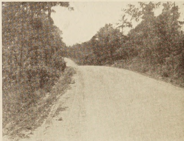
SHOULDER MATERIAL BLADED OVER WEAK PAVEMENT EDGE IN SOUTH CAROLINA
