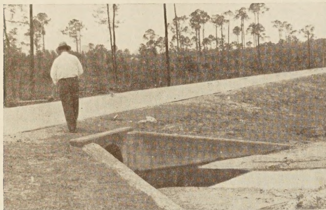
SURFACE TREATED SAND-CLAY ROAD WITH CYPRESS CURBS AND WIDE SLOPING SHOULDERS ON SECTION 1 IN FLORIDA
