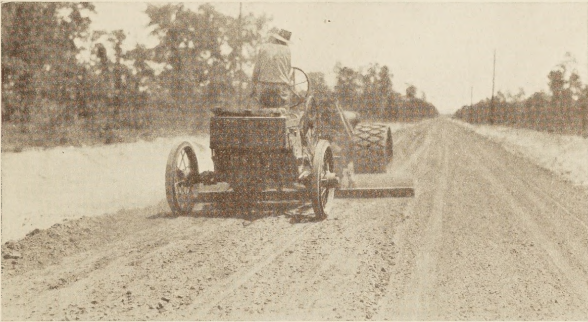
PREPARING A SAND-CLAY ROAD FOR SURFACE TREATMENT
