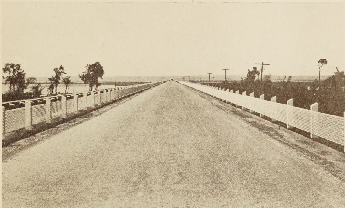
BITUMINOUS SURFACE TREATED SAND-CLAY ROAD. SECTION 1 IN FLORIDA BETWEEN PENSACOLA AND TALLAHASSEE
