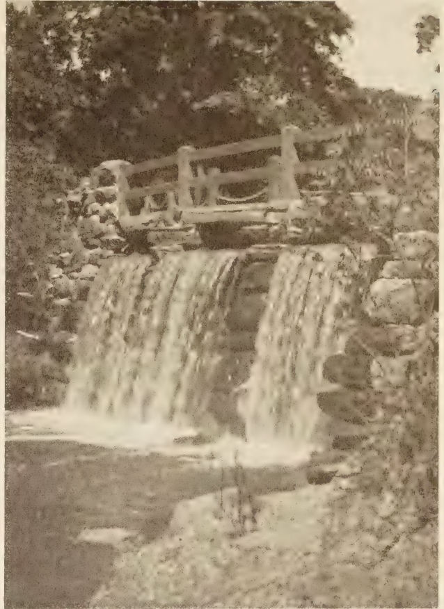
A FOOTBRIDGE AND SPILLWAY ON TIBBITS BROOK, WEST-CHESTER COUNTY, N. Y.
