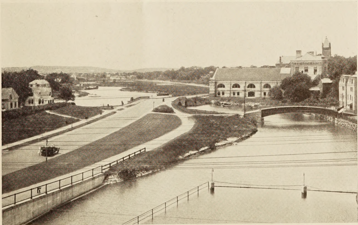
PARKWAYS CONSTRUCTED BY THE PARKS DIVISION OF THE METROPOLITAN DISTRICT COMMISSION OF MASSACHUSETTS. UPPER—WOBURN PARKWAY NEAR WOBURN. LOWER—MYSTIC VALLEY PARKWAY NEAR MEDFORD
