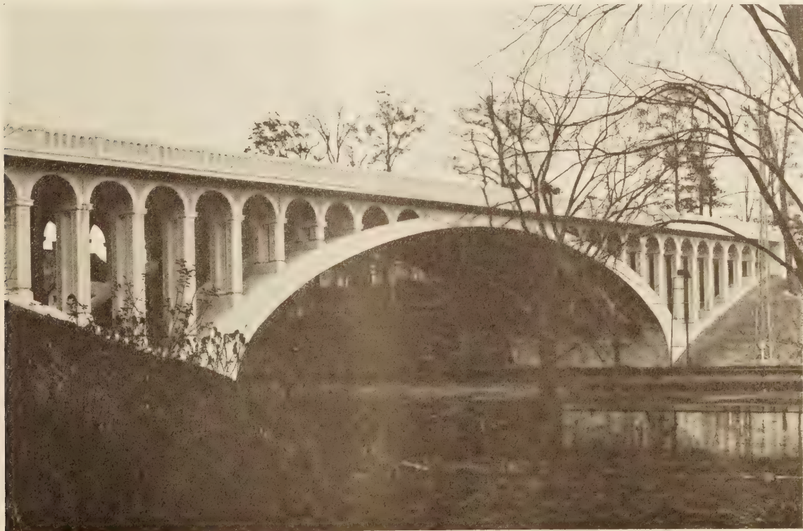
REINFORCED CONCRETE BRIDGE, BRONX RIVER PARKWAY, NEW YORK
