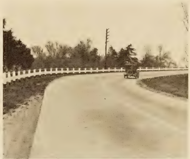
A WIDENED AND SUPERELEVATED CURVE
