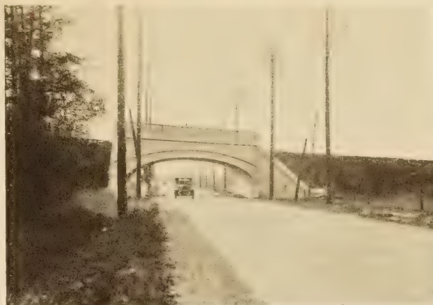
RAILROAD GRADE CROSSING ELIMINATION
