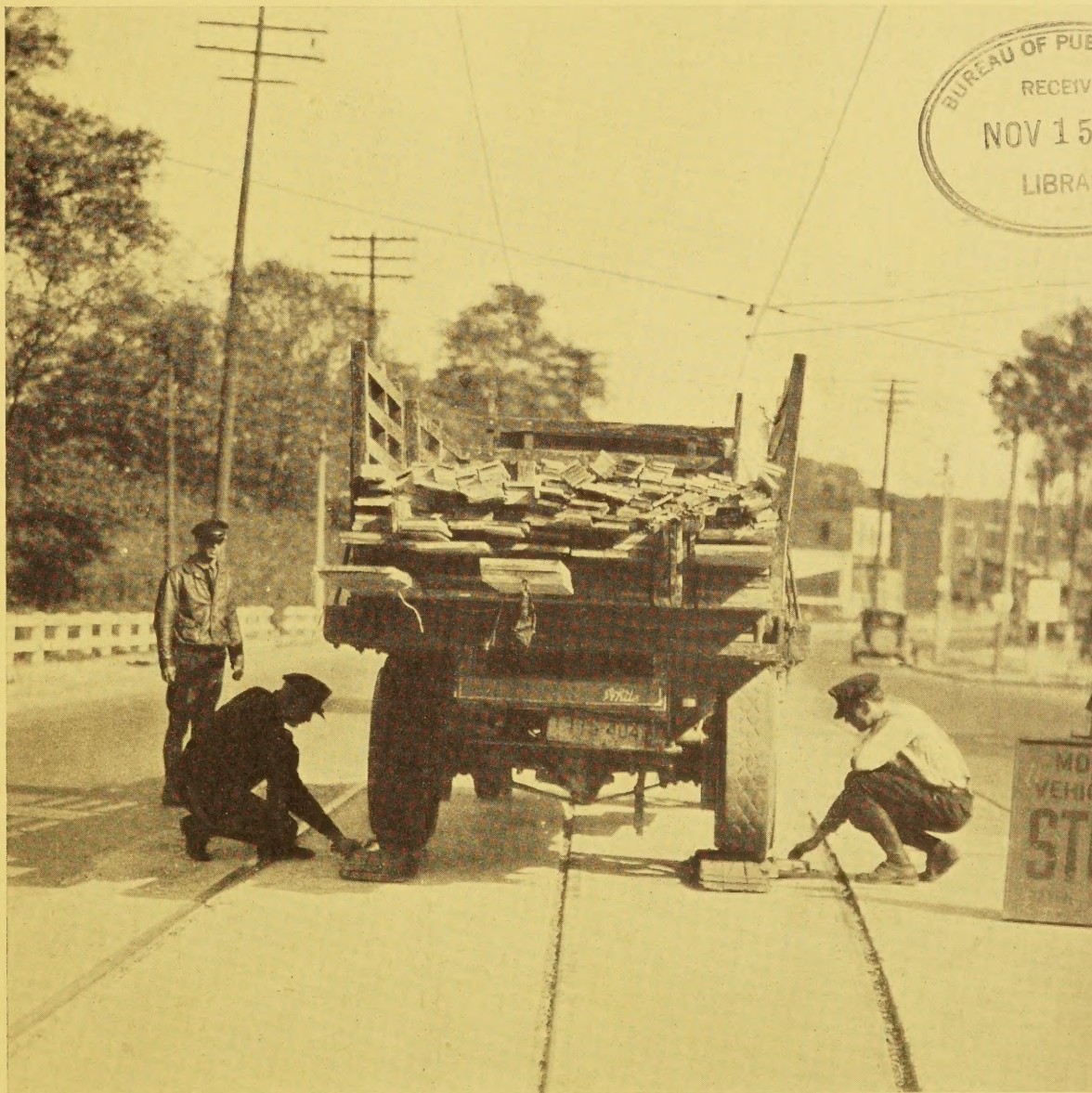
WEIGHING A TRUCK AT A TRAFFIC SURVEY STATION
