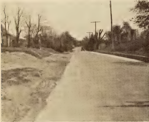
PRESENT CONDITION OF BRADLEY LANE AT A POINT WHERE DRAINAGE IS TOWARD THE ROAD FROM BOTH SIDES
