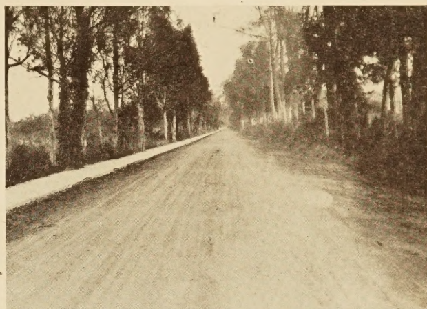
CONDITION OF SURFACE AFTER SURFACE TREATMENT IN 1911
