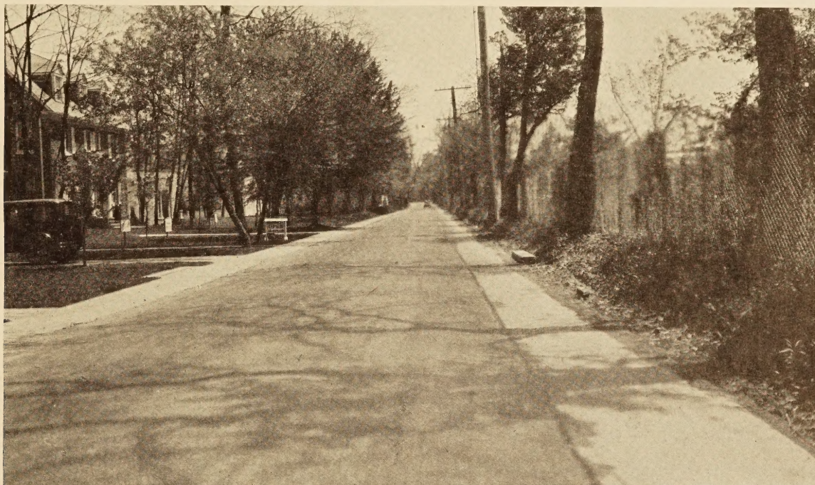
PRESENT CONDITION OF BRADLEY LANE. THE DRAINAGE ON THE LEFT IS TOWARD THE ROAD SURFACE
