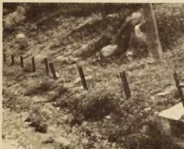
STEEL RAILS USED TO HOLD A SLIDE
