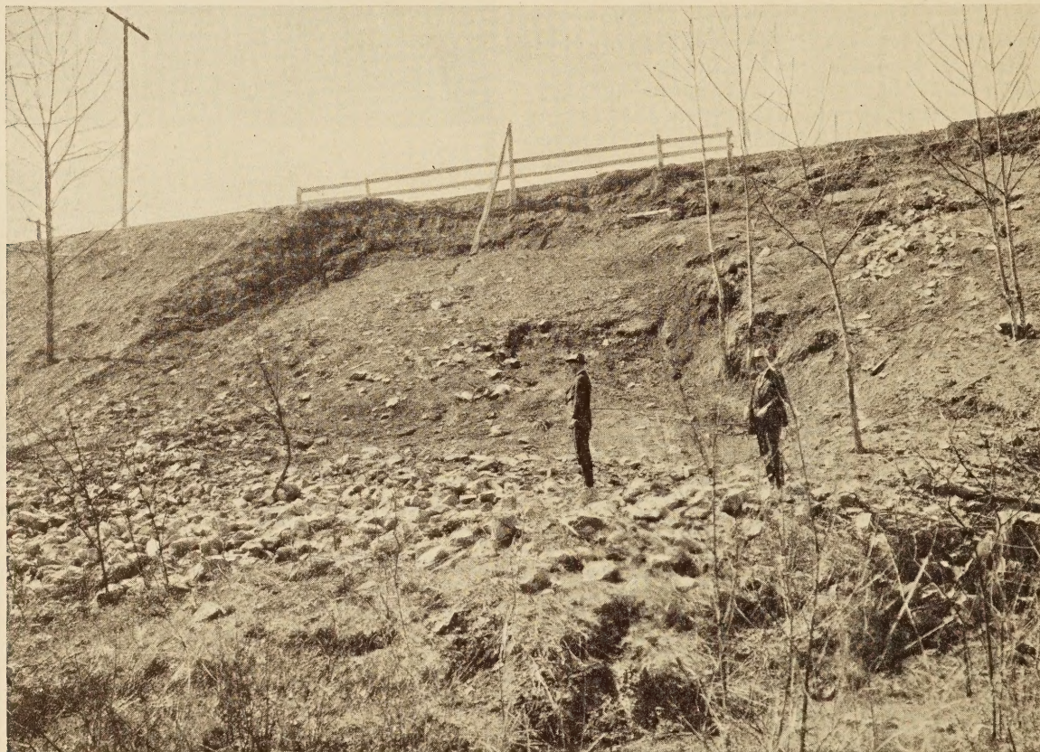
FILL SLIDE AT LEE'S CREEK, W. VA.
