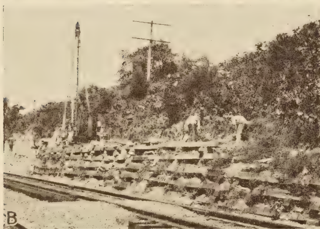
TIMBER CRIBBING FOR SLIDE CONTROL
