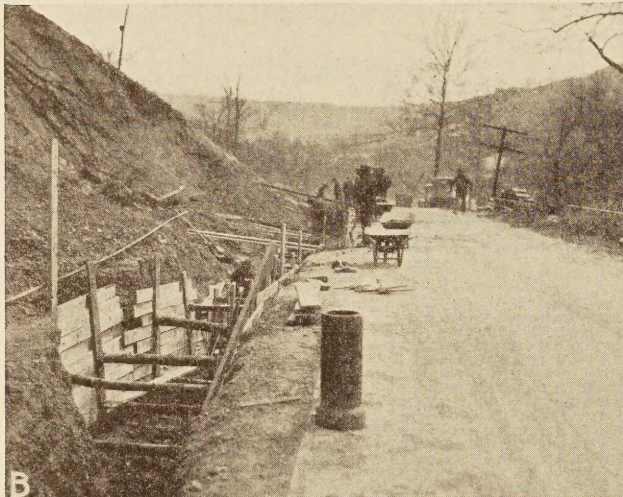
A CONCRETE ROAD SUPPORTED ON POSTS AFTER A SIDEHILL SLIDE
