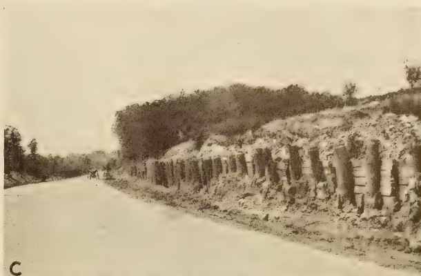
TYPES OF RETAINING WALL USED TO PROTECT ROAD
