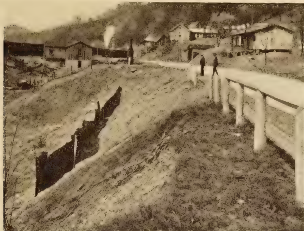
SHEET PILING USED TO HOLD A FILL
