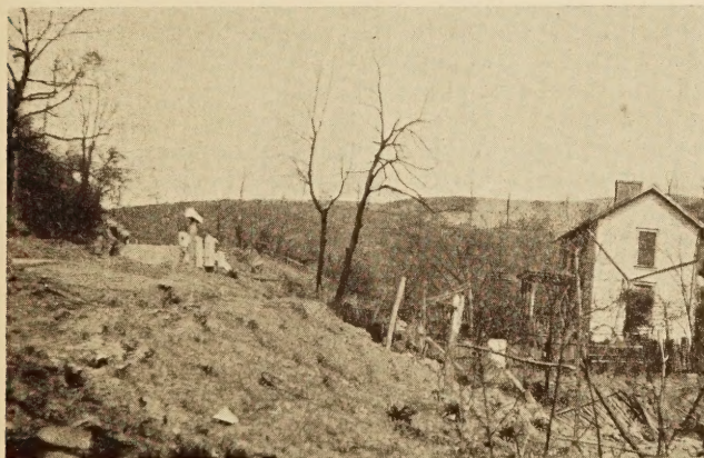
AN OLD SLIDE STARTED IN MOTION BY WEIGHT OF NEW HIGHWAY FILL OF ONLY MODERATE HEIGHT
