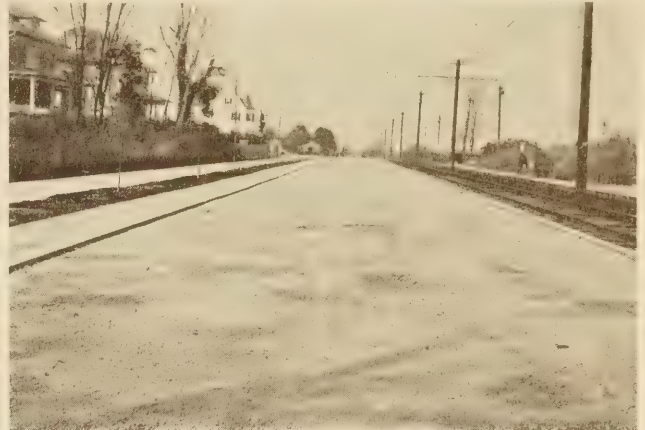
CONCRETE BASE FOR ASPHALTIC CONCRETE SECTIONS
