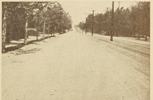
STEPS IN CONSTRUCTION AND FINISHED PAVEMENT OF PENETRATION MACADAM, EXPERIMENT 3
