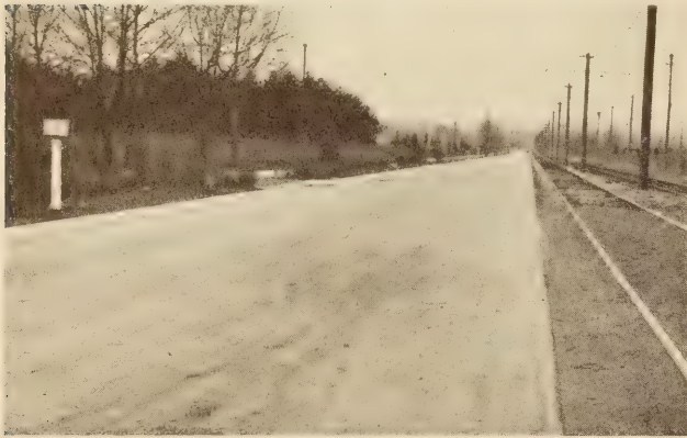
CONDITION OF 2 OF THE SURFACE-TREATED PORTLAND CEMENT CONCRETE SECTIONS IN 1914
