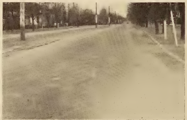
CONDITION OF EXPERIMENT 11 IN FEBRUARY, 1928. WATER-BOUND MACADAM SURFACE TREATED WITH ASPHALT EMULSION
