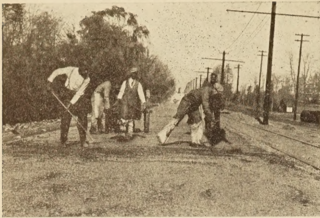
HAND POURING THE SEAL COAT ON ONE OF THE PENETRATION MACADAM SECTIONS
