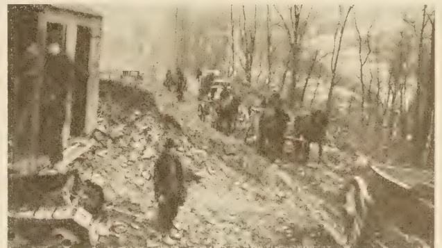
"BOTTLE NECKS" ALMOST ALWAYS INCREASE THE AVERAGE TRIP TIME OF HAULING UNITS
