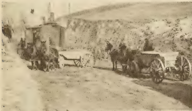
TYPICAL OPERATION WITH TEAM HAULING
