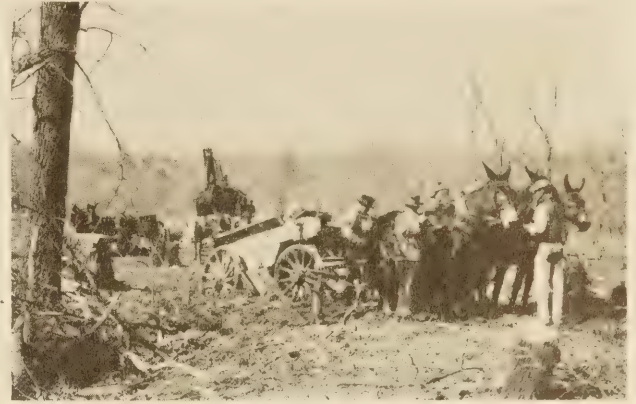
LIGHT LOADS AND INCREASED HAULING TIME CAUSED BY STUMPS AND SOFT GROUND
