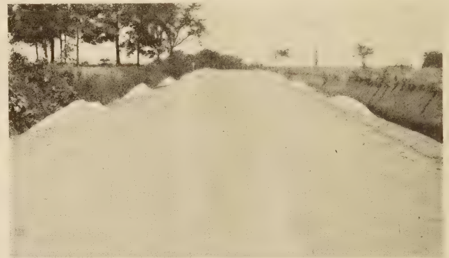
A WELL BONDED TOPSOIL SURFACE SUITABLE FOR DOUBLE SURFACE TREATMENT
