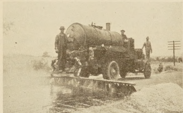
APPLYING PRIMING COAT TO THE TOPSOIL SURFACE
