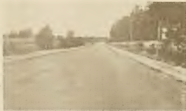
TAR MIXED SECTION WITHOUT SEAL COAT SHORTLY AFTER CONSTRUCTION
