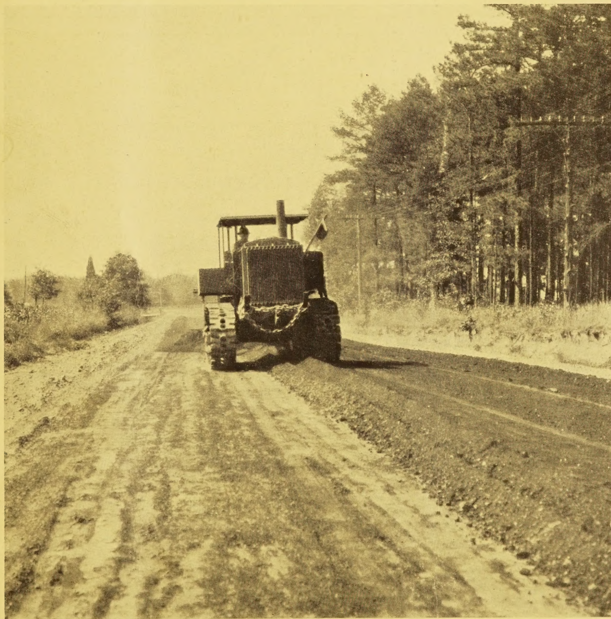
MIXING TOPSOIL WITH BITUMINOUS MATERIAL IN SOUTH CAROLINA EXPERIMENTS
