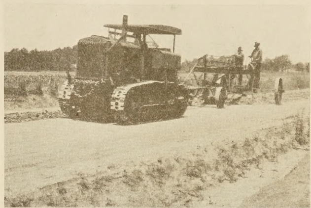
SCARIFYING TOPSOIL SURFACE FOR THE MIXING TREATMENT
