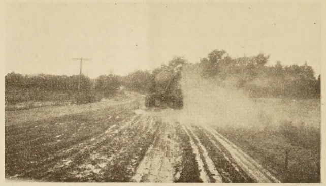
FINAL APPLICATION OF BITUMINOUS MATERIAL PREPARATORY TO MIXING
