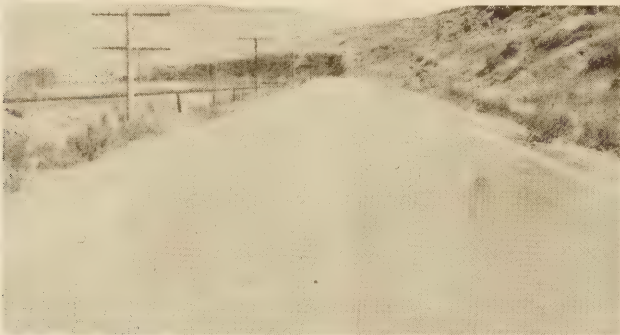
FIG. 7.—MILE 106 ON THE COLUMBIA RIVER HIGHWAY. SURFACED IN 1921, RESURFACED AND OILED IN 1924, AND REOILED IN 1925
