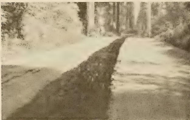
FIG. 26.—MULCHING PARTLY BLADED BACK OVER OILED SURFACE
