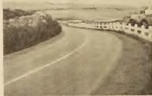
FIG. 17.—MILE 206 ON COLUMBIA RIVER HIGHWAY. RESURFACED IN 1924 AND TREATED WITH OIL AT A RATE OF 0.495 GALLON PER SQUARE YARD IN 1925. NOTE THE TRAFFIC GUIDE LINE AS USED UPON HIGH-TYPE SURFACES
