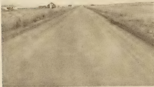
FIG. 15.—MILE 166 ON THE COLUMBIA RIVER HIGHWAY. RESURFACED IN 1923. TREATED WITH OIL AT A RATE OF 0.495 GALLON PER SQUARE YARD AND STONE SCREENINGS AT A RATE OF 15 TO 20 CUBIC YARDS PER MILE IN 1925
