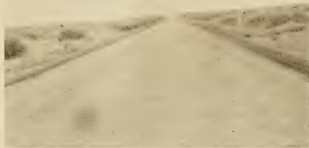
FIG. 12.—MILE 176 ON COLUMBIA RIVER HIGHWAY. RE-SURFACED IN 1923 AND OILED IN 1925
