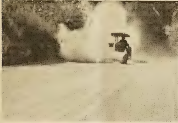
FIG. 23.—POWER BROOM ATTACHED TO FRONT END OF A TRACTOR USED FOR CLEANING SURFACE BEFORE APPLICATION OF OIL
