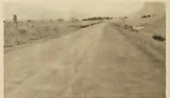
FIG. 9.—MILE 126 ON COLUMBIA RIVER HIGHWAY. RESURFACED WITH CRUSHED ROCK BOUND WITH CLAY IN 1924. OIL APPLIED AT A RATE OF 0.5 GALLON PER SQUARE YARD TO UNSWEPT SURFACE IN 1925. SURFACE IS NOT ROUGH BUT LACKS UNIFORMITY
