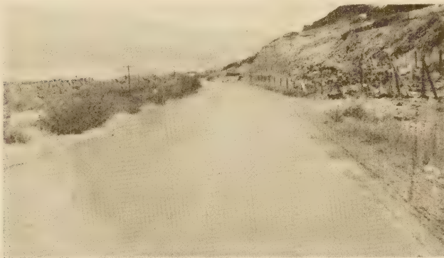
FIG. 6.—MILE 96 ON COLUMBIA RIVER HIGHWAY. SURFACED IN 1921, RESURFACED AND OILED IN 1924
