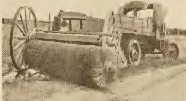
FIG. 2.—POWER BROOM FOR CLEANING ROAD SURFACE PRIOR TO TREATMENT
