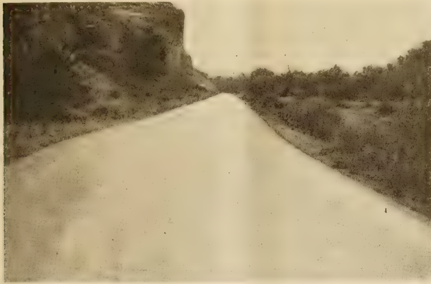
FIG. 18.—MILE 216 ON COLUMBIA RIVER HIGHWAY. RE-SURFACED IN 1923 AND OILED IN 1925
