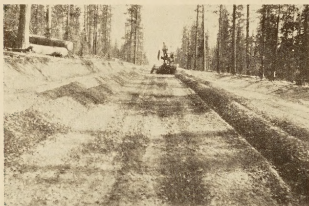
FIG. 1.—MIXING ROAD METAL AND BINDER, ONE OF THE PROCESSES IN THE CONSTRUCTION OF FINE CRUSHED ROCK AND GRAVEL ROADS
