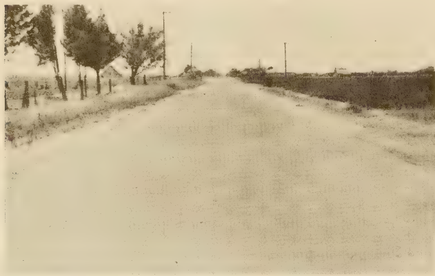
FIG. 33.—TYPICAL SECTION OF THE TURLOCK-SNELLING ROAD. THE SANDY SOIL IS PROBABLY RESPONSIBLE FOR THE SUCCESS OF THE ROAD IN SPITE OF LACK OF DRAINAGE
