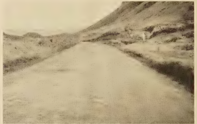
FIG. 8.—MILE 116 ON COLUMBIA RIVER HIGHWAY. SURFACED WITH CRUSHED GRAVEL BOUND WITH CLAY IN 1924. LOOSE UNSWEPT SURFACE TREATED WITH 0.24 GALLON PER SQUARE YARD IN 1924. REOILED IN 1925 AT A RATE OF 0.42 GALLON PER SQUARE YARD
