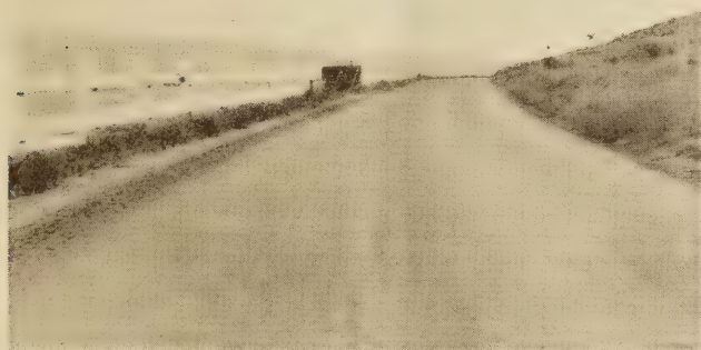
FIG. 11.—MILE 146 ON COLUMBIA RIVER HIGHWAY. RE-SURFACED WITH CRUSHED CEMENTITIOUS GRAVEL IN 1925. OILED IN THE SPRING OF 1926
