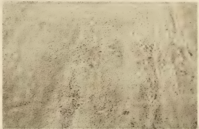
FIG. 24.—EXPOSED ROCK SURFACE UPON COMPLETION OF BROOMING
