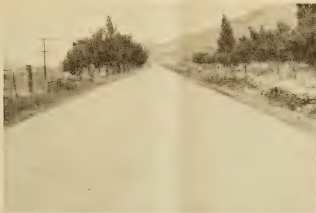
FIG. 10.—MILE 136 ON COLUMBIA RIVER HIGHWAY. RE-SURFACED IN 1924, USING CEMENTITIOUS GRAVEL FOR SURFACE COURSE. OIL APPLIED IN 1925 AT A RATE OF 0.5 GALLON PER SQUARE YARD. THE SURFACE IS UNIFORMLY SMOOTH
