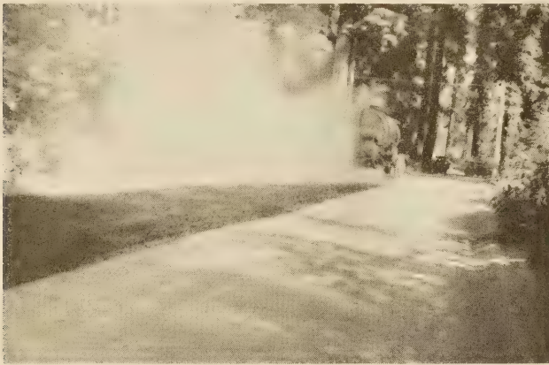
FIG. 25.—APPLICATION OF OIL TO CLEANED SURFACE
