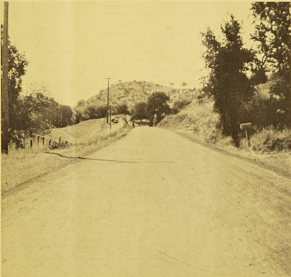
A CALIFORNIA HIGHWAY TREATED WITH LIGHT ASPHALTIC OIL
