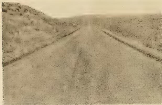
FIG. 14.—MILE 156 OF COLUMBIA RIVER HIGHWAY. RESURFACED WITH CRUSHED CEMENTITIOUS GRAVEL IN 1925 AND TREATED WITH 0.5 GALLON PER SQUARE YARD OF OIL IN THE SPRING OF 1926
