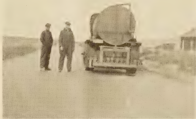
FIG. 3.—TYPE OF DISTRIBUTOR USED FOR APPLICATION OF OIL
