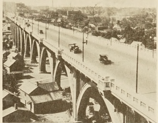
NORTH HILL VIADUCT AT AKRON, OHIO. LENGTH 2,800 FEET; ROADWAY, 52 FEET; BUILT 1921
