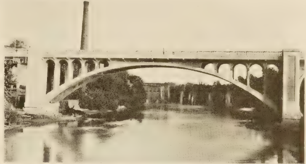
A TWO-RIBBED OPEN-SPANDREL ARCH DESIGNED BY THE METHOD DESCRIBED HERE BUT WITH SOME VARIATION ON ACCOUNT OF THE POSITION OF LOAD POINTS AS FIXED BY THE LOCATION OF COLUMNS
