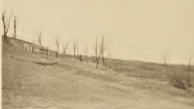
FIG. 21.—TYPICAL FILL SLIDES. IN THE LOWER PICTURE A NATURAL SLIDE IS TO BE SEEN IN THE FIELD BELOW THE FILL SLIDE
