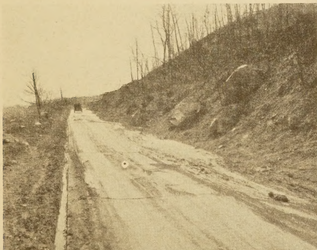
FIG. 1.—DAMAGE TO A HIGHWAY BY A LANDSLIDE RESULTING IN SUBSIDENCE, UPHEAVAL, AND LATERAL DISLOCATION
