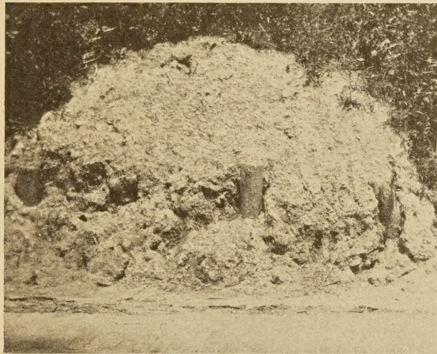
FIG. 10.—DETRITAL SLIDE MOVING THROUGH PILES AND SHOWING FLOW CHARACTERISTICS VERY PLAINLY. THIS SLIDE OCCURRED IN OHIO WHERE THE DETRITUS CONTAINS MORE CLAY AND LESS SANDSTONE THAN IN WEST VIRGINIA
