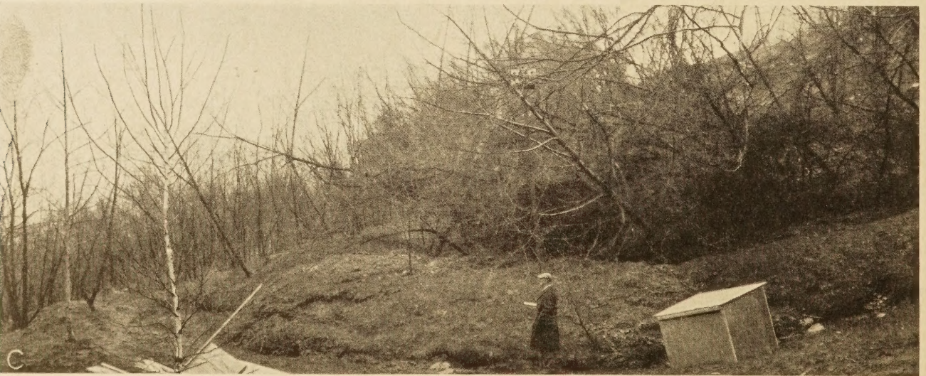
FIG. 12.—VIEWS OF THE TOP, MIDDLE, AND BOTTOM OF A LANDSLIDE NEAR HUNTINGTON, W. VA., ARRANGED IN THE ORDER MENTIONED. NOTE THE BEGINNING OF A BREAK AND THE OLD SLIDE IN THE TOP PICTURE, THE FLUID CHARACTER OF MATERIAL IN THE CENTER PICTURE AND THE UPHEAVAL OF MATERIAL AT THE BOTTOM DUE TO IMPACT OF THE SLIDE
