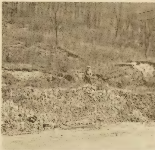
FIG. 13.—FISSURES AND POCKETS ARE TYPICAL OF DETRITAL SLIDES. THEY CATCH SURFACE WATER AND ARE OFTEN FACTORS IN KEEPING THE SLIDE MOVING
