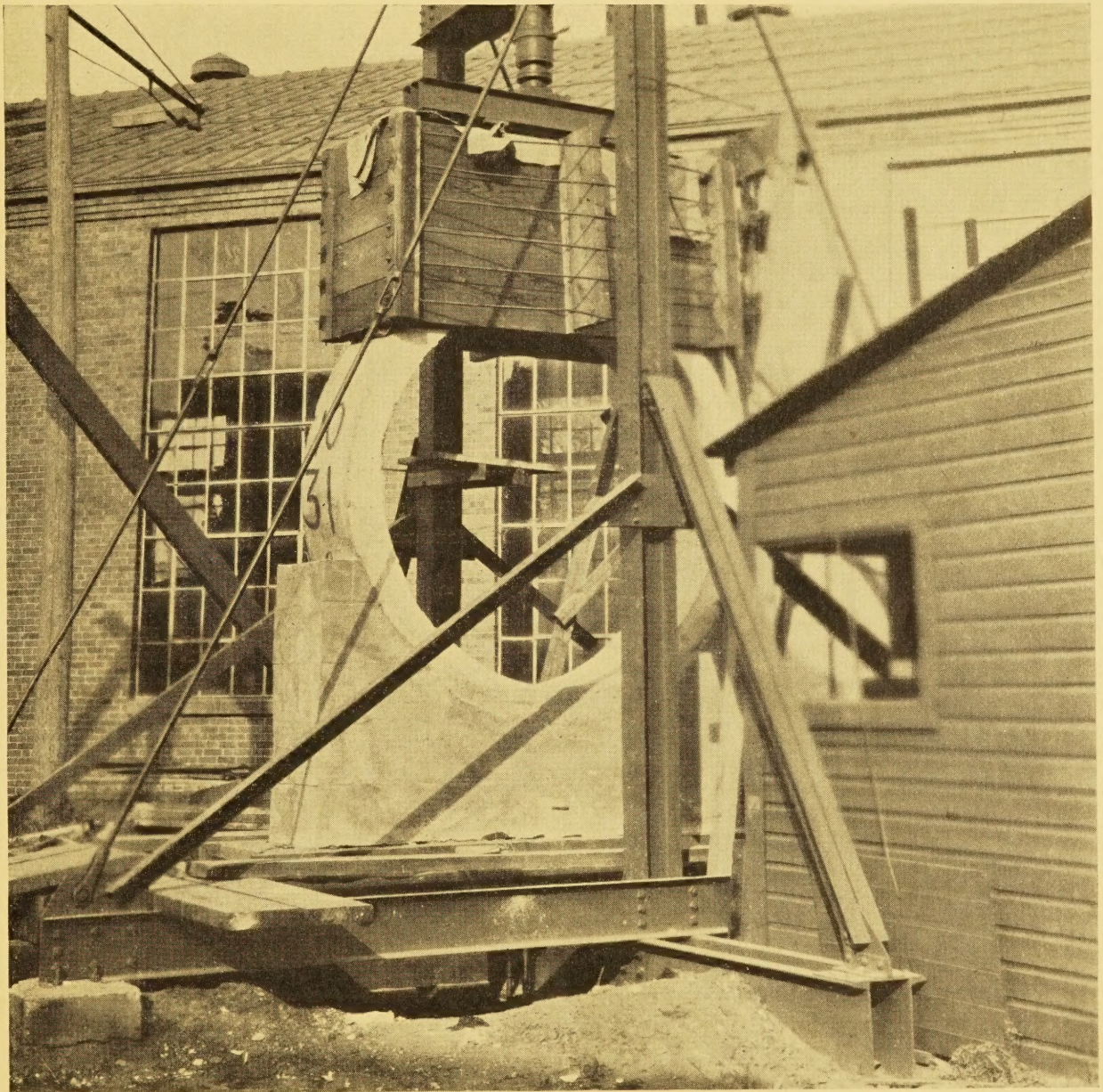
APPARATUS USED FOR IOWA PIPE TESTS
