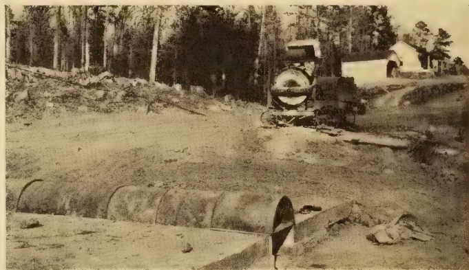
TEST PIPE IN PLACE
