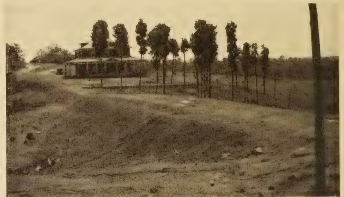
FILL AT CHAPEL HILL, N. C., AT END OF TIME AND WEATHER TEST
