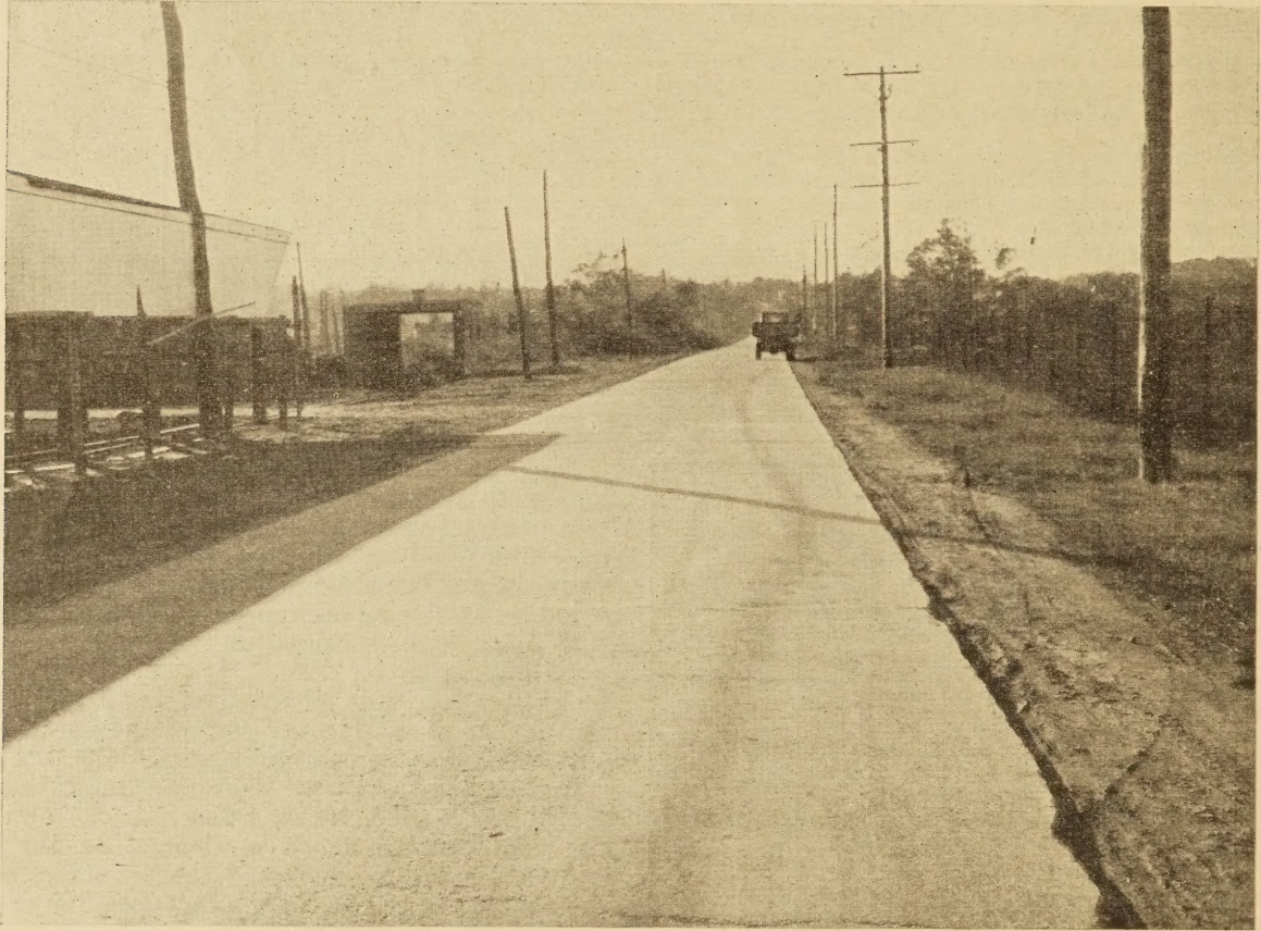
FIG. 10.—The smooth concrete test section
