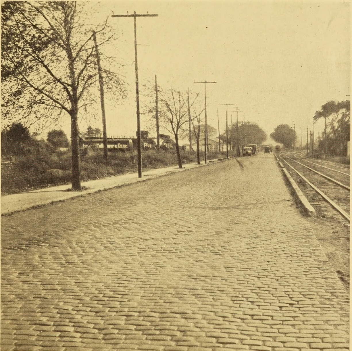
THE ROUGH STONE BLOCK TEST HIGHWAY USED IN THE IMPACT TESTS
