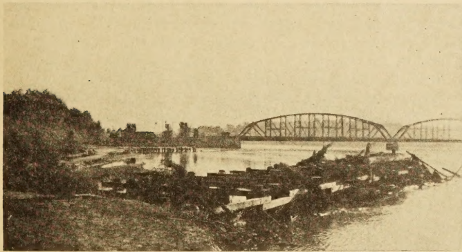
FIG. 3.—Middle dike of a series of three pile dikes protecting bridge at Leavenworth Kans. Note accumulation of drift
