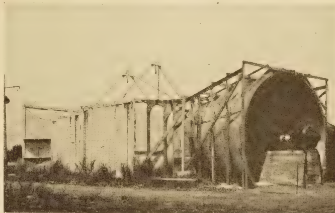
FIG. 1.—The tunnel used in the wind-resistance tests
