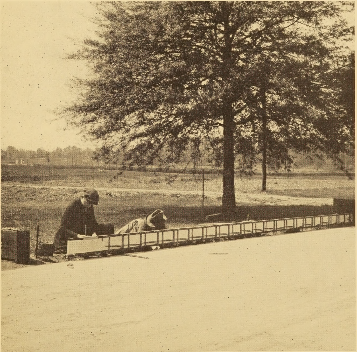
GENERAL VIEW OF DEFLECTOMETER USED IN TESTS OF SIX-WHEEL TRUCKS
