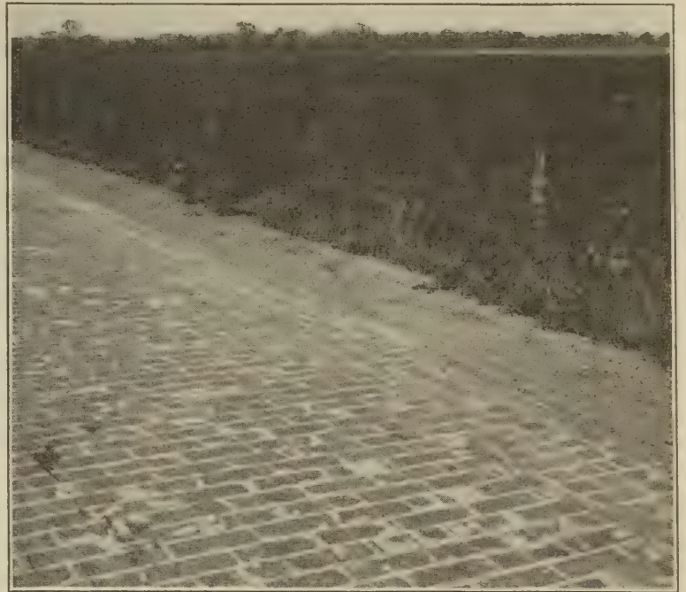
FIG. 1.—GROUT FILLED BRICK PAVEMENT ON GRAVEL BASE, COLUMBUS-CHILlicothe ROAD.
