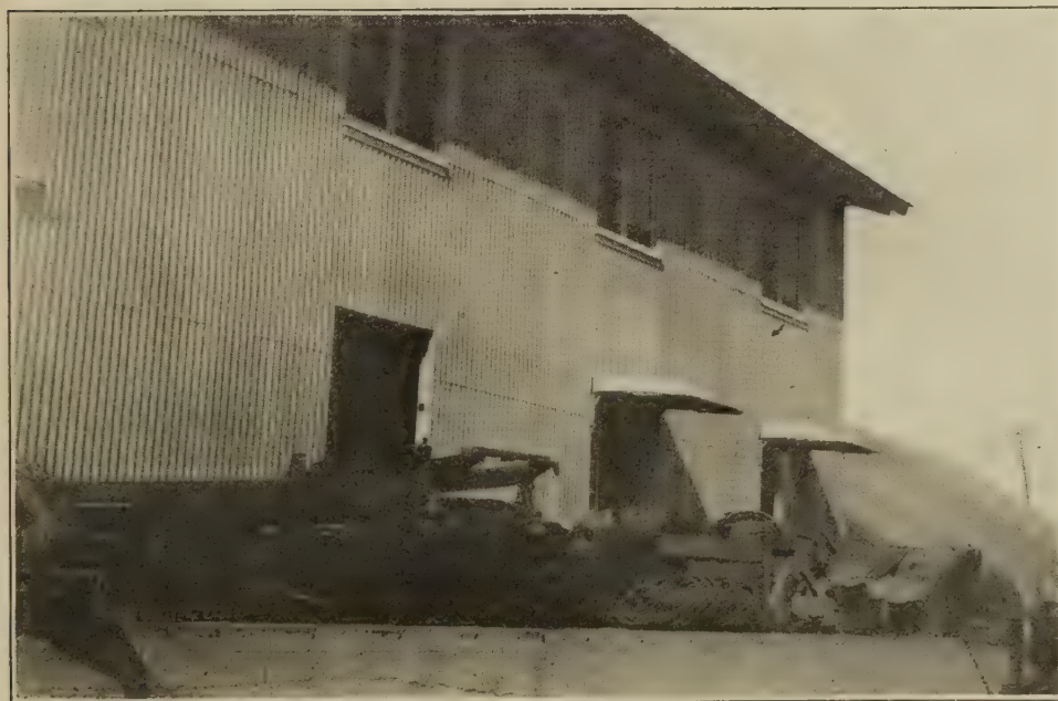
A WAREHOUSE FOR WAR MATERIALS IN ARIZONA, BUILT WITH GOVERNMENT MATERIAL. NOTE THE TRUCK SEAT TOPS USED AS AWNINGS.
