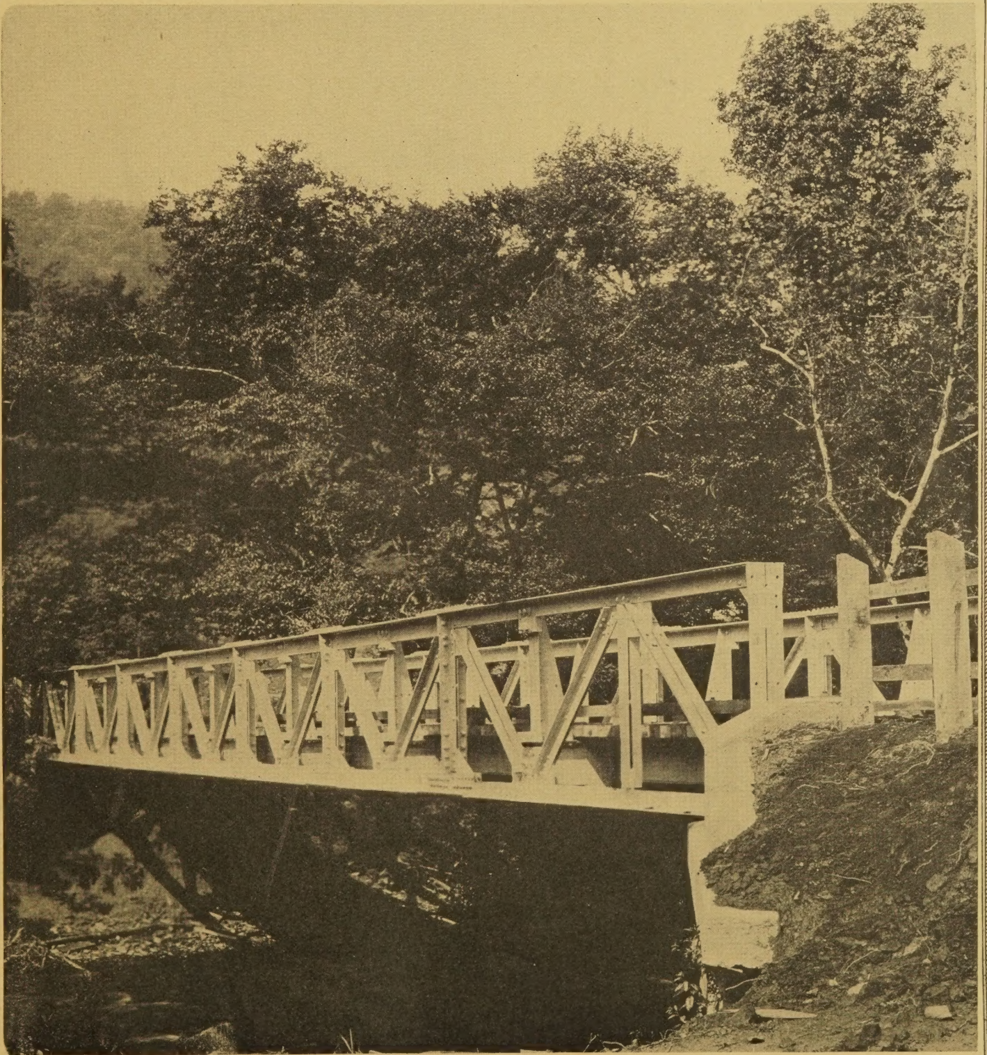
ARMY SECTIONAL BRIDGE ERECTED OVER DAVIDSON RIVER, PISGAH NATIONAL FOREST
