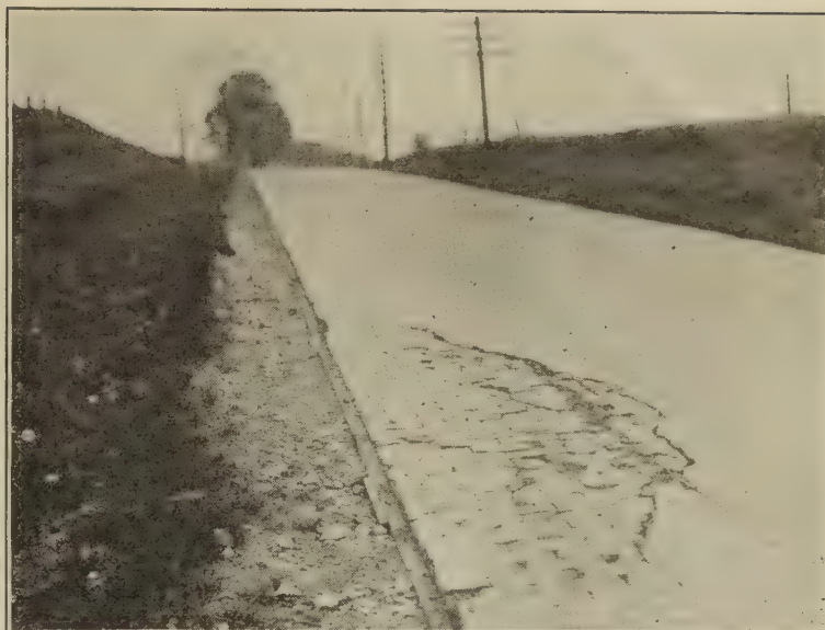
FIG. 5.—GROUTED BRICK ROAD ON SLAG BASE, MAHONING COUNTY, OHIO.
