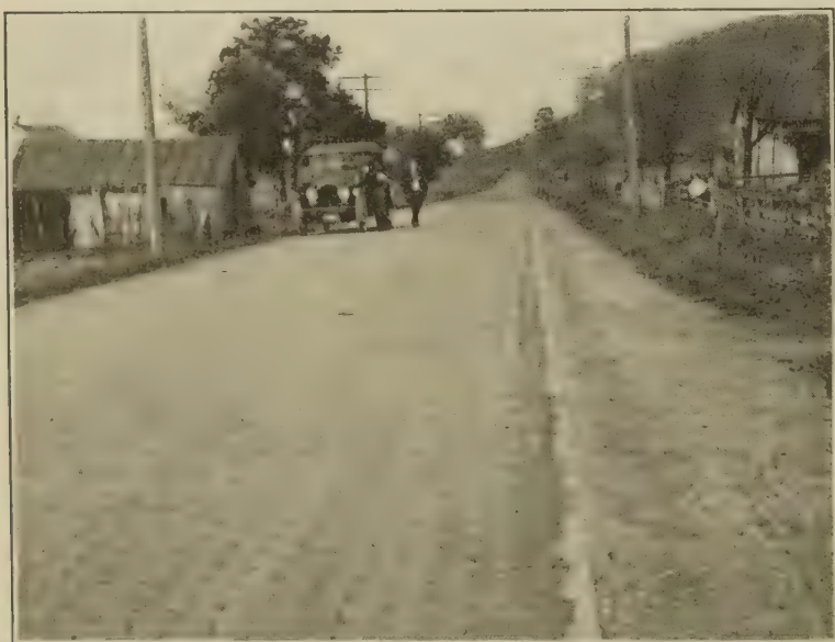
FIG. 2.—BRICK ROAD ON GRAVEL BASE, TAR-MASTIC FILLER.
