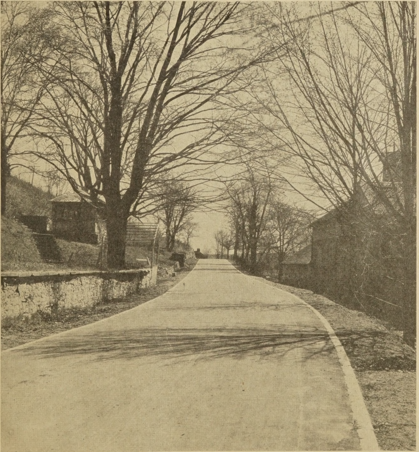
PENNSYLVANIA FEDERAL-AID PROJECT NO. 29—AN ASPHALT CONCRETE ROAD
