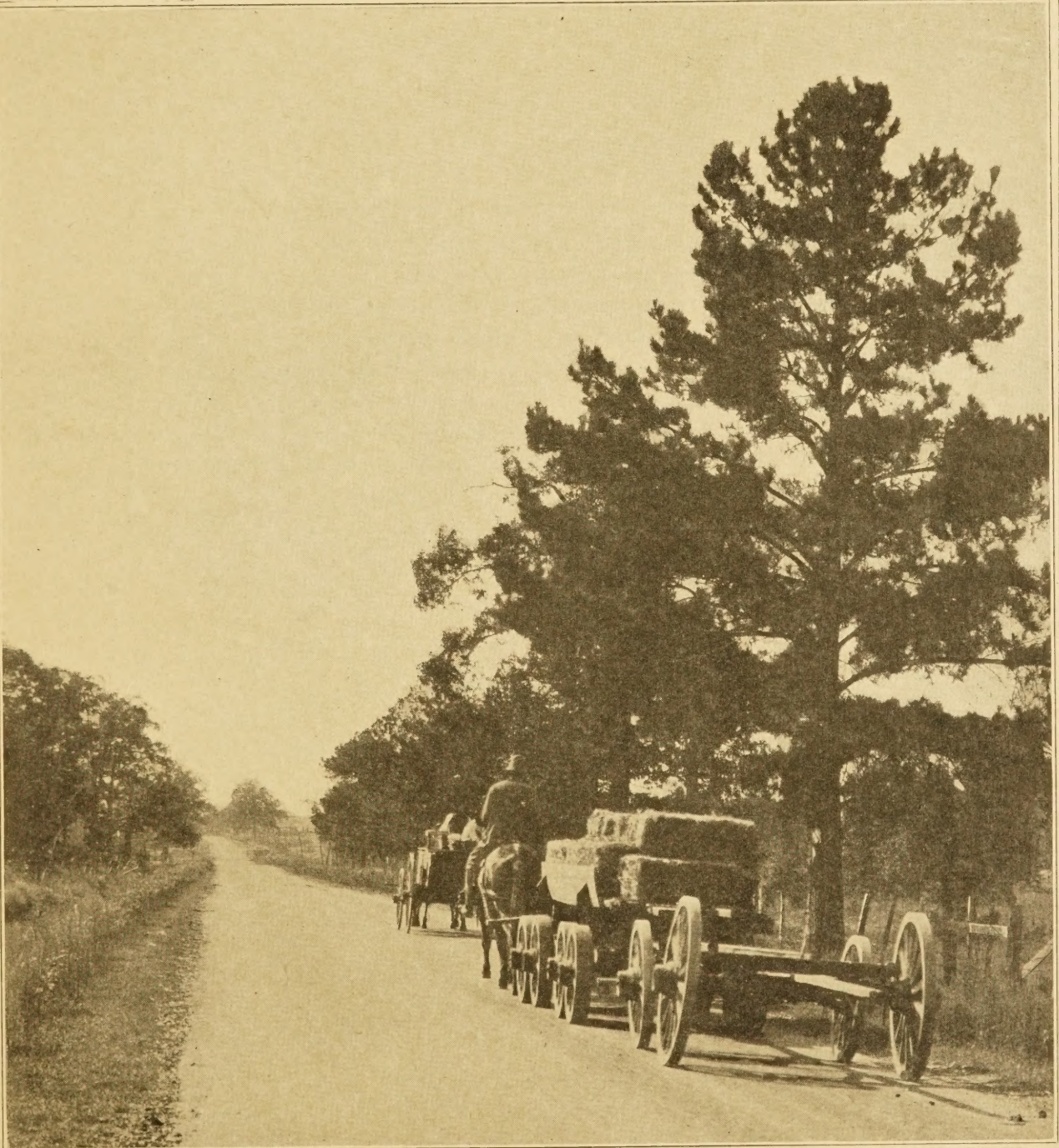
TEXAS FEDERAL-AID PROJECT NO. 21, FROM GLADEWATER TO LONGVIEW
