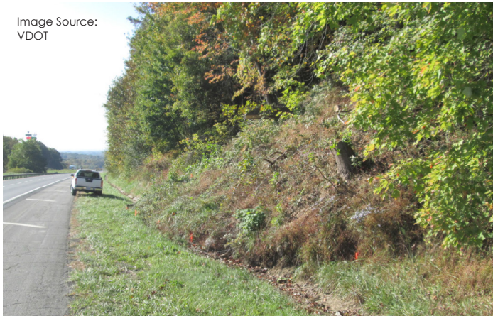
Figure 2: Soil slope slide along I-77.
