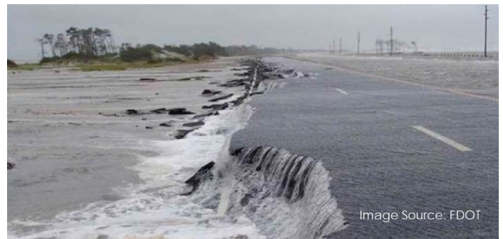
Figure 4: US 98 damage to the north pavement edge during a 2005 tropical storm (prior to the 2006 installation of protection measures).
