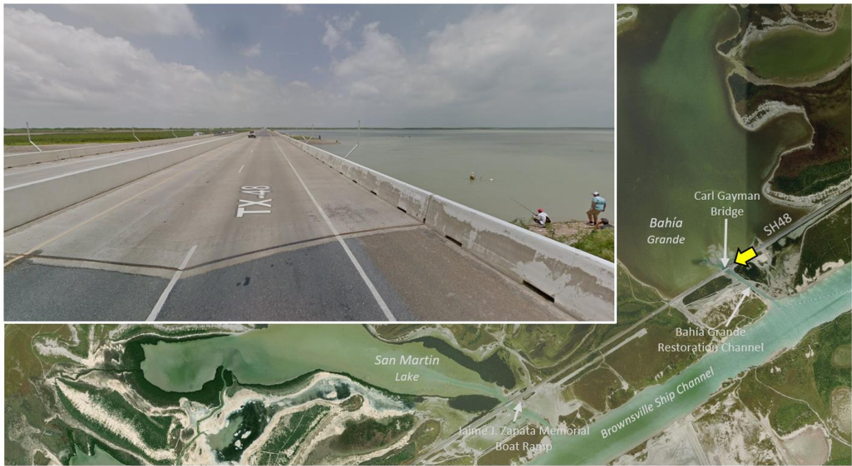
Figure 7. Google Street View of Westbound SH 48 Just East of the Carl Gayman Bridge over the Bahía Grande Restoration Channel. Bahía Grande is on the right. The view shows the 48-inch-high center CTB, and the 36-inch-high north (right) and south (far left) outer traffic barriers. The 12-foot high, barrier-mounted pelican poles are visible on both sides of the bridge. The yellow arrow on the map indicates approximate photo location and direction (image captured June 2019).
