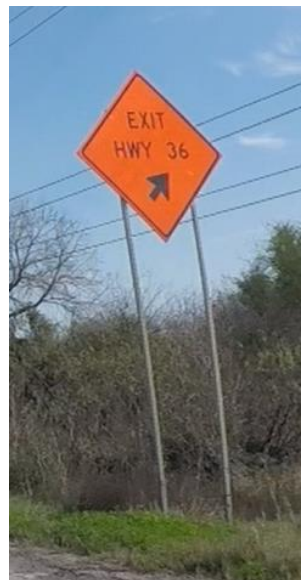
(b) Exit direction sign
