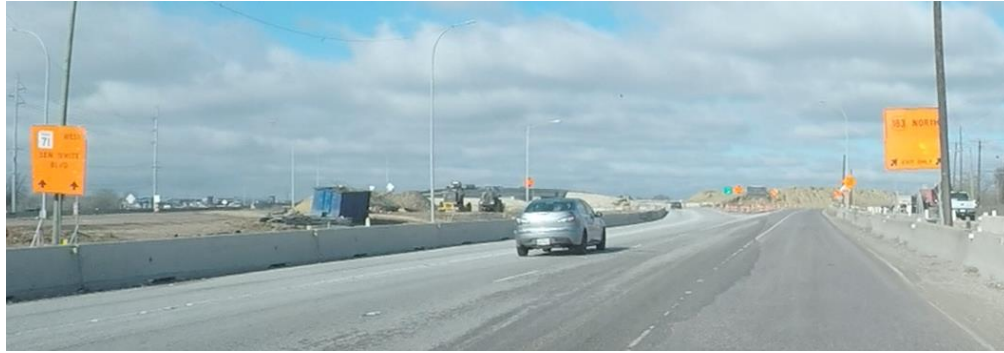
Figure 16. Temporary Lane Guidance Signs at Interchange Exit.
