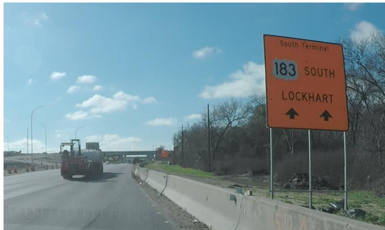
Figure 15. Temporary Lane Guidance Sign with Up Arrows Used on Roadside.
