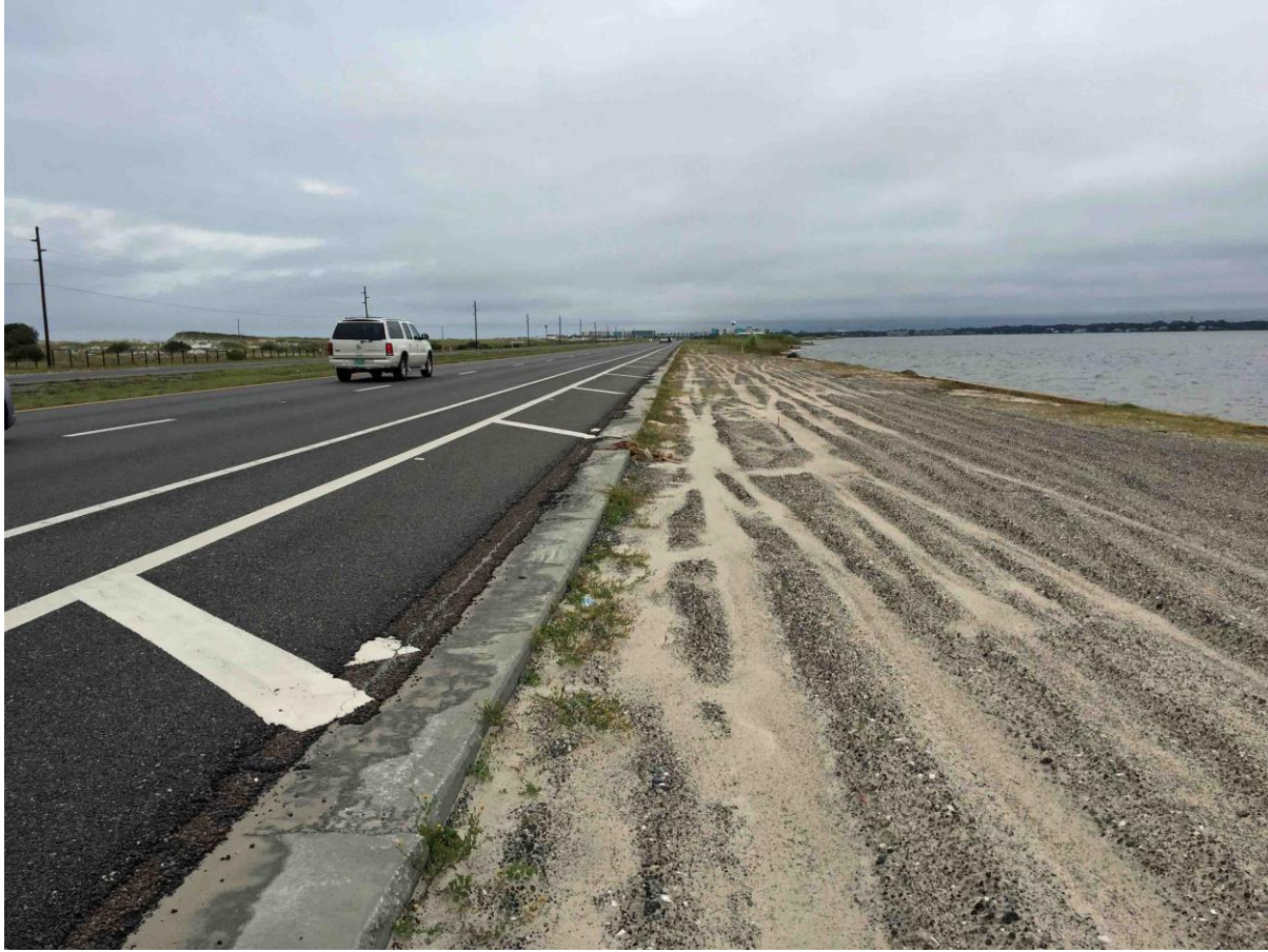
Figure 9: Photograph showing the top of concrete pile cap (left side of photograph) on the buried 18-foot deep sheet pile wall protecting the north side of the eastbound travel lanes on US 98 between Destin Pass and Okaloosa Island. Note that there is a buried gabion mat (not visible) below the location of the photographer. 23
