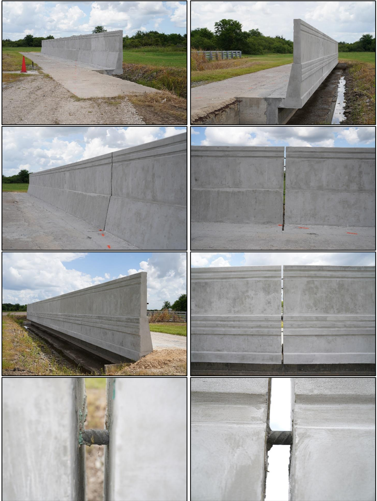
Figure 2.2. TxDOT T80SS Barrier with Soundwall prior to Testing.
