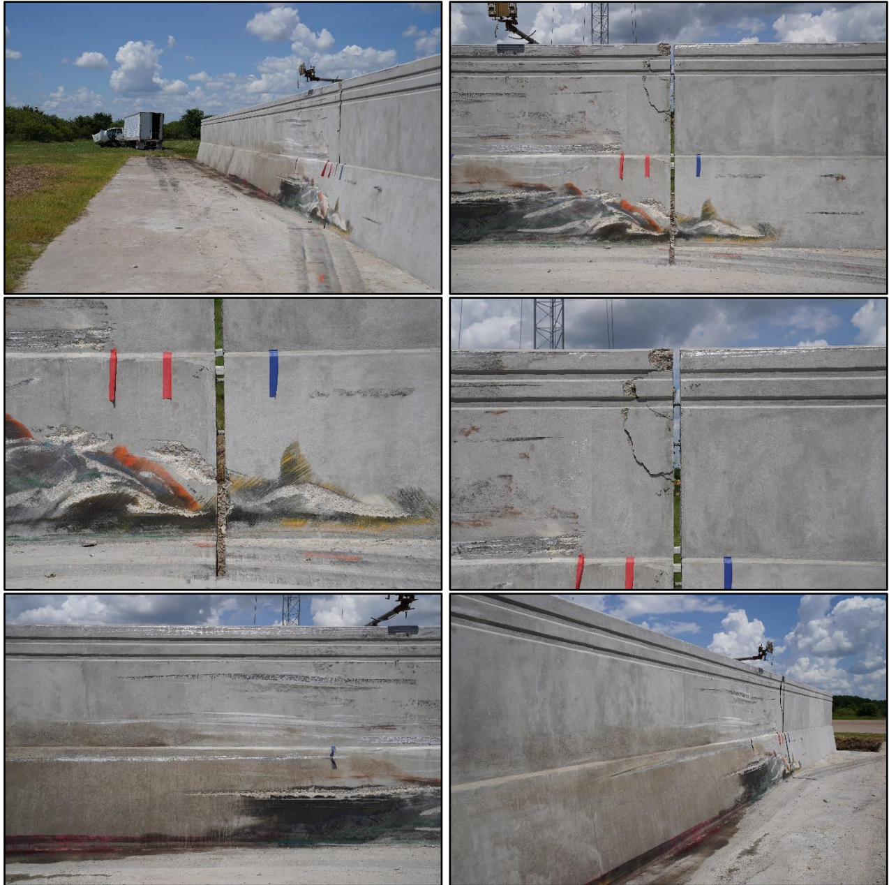
Figure 5.3. TxDOT T80SS Barrier with Soundwall after Test No. 440861-4.
