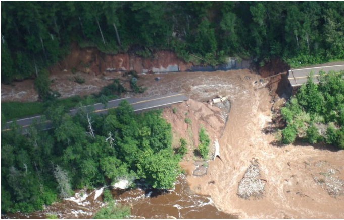
Figure 1. A highway in Minnesota is washed out due to flooding from a mega-rain event. Photo credit: MnDOT.
