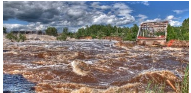
Figure 2. Flood waters washing out a road and bridge in District 1. Photo credit: MnDOT.
