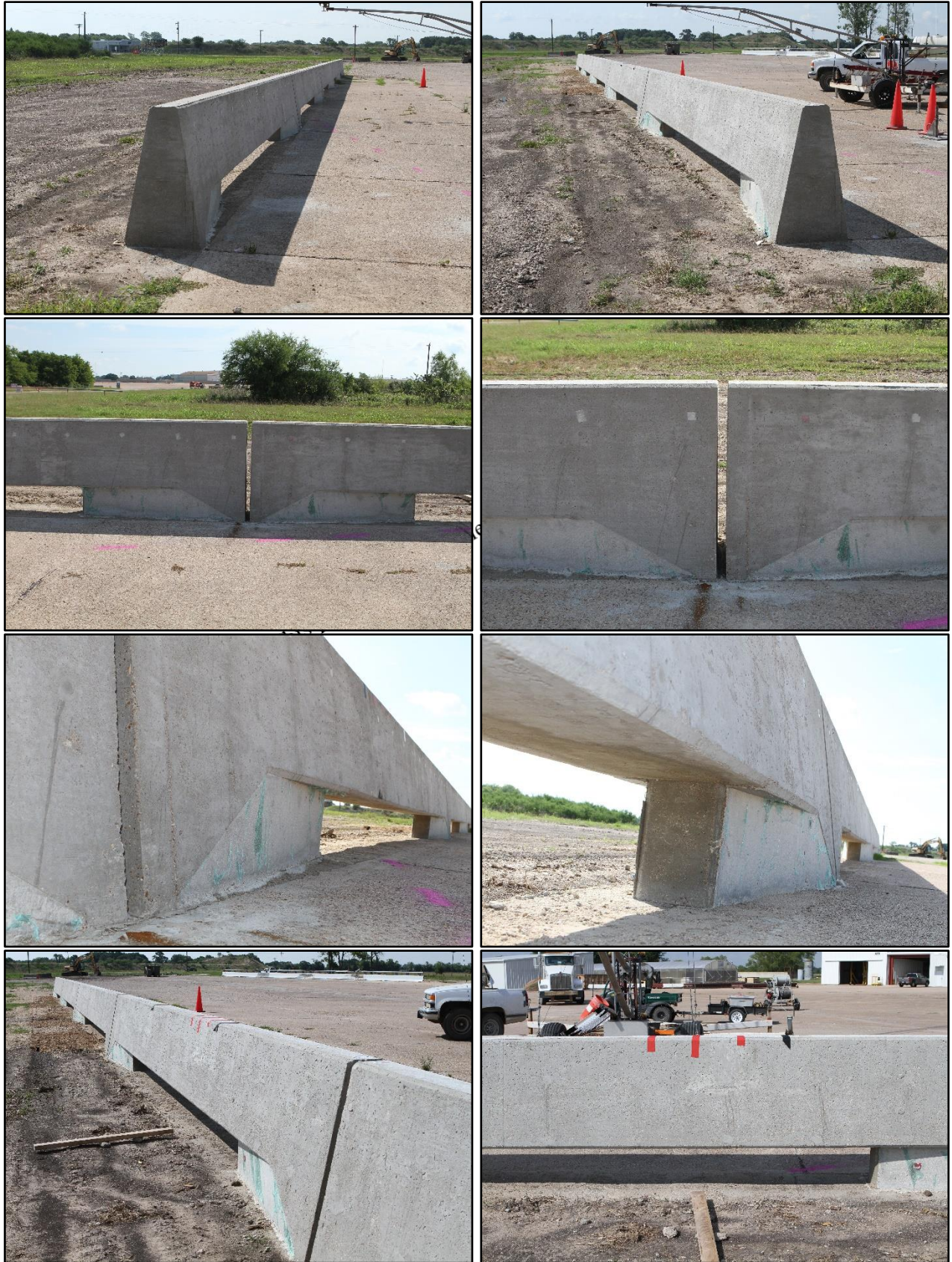
Figure 6.2. TxDOT LSMB prior to Testing.
