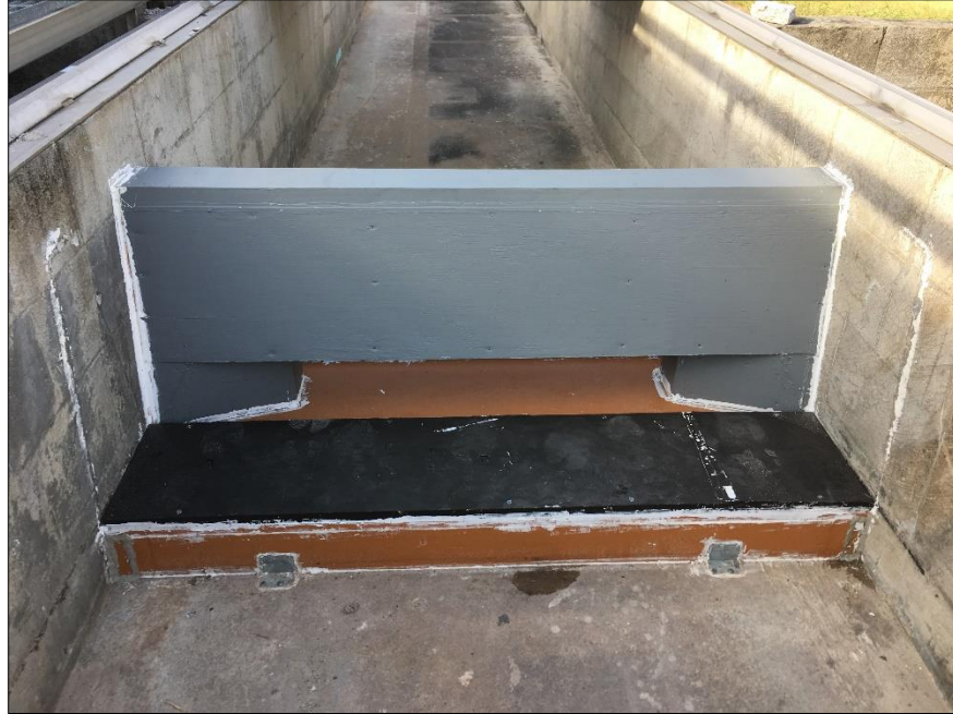
Figure 5.16. SSCB with Overlay.
