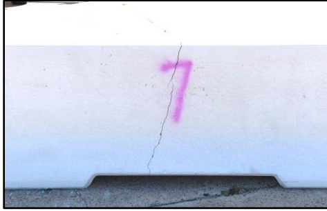
Figure 2.19. Concrete Crack after MASH Test 2-11.
