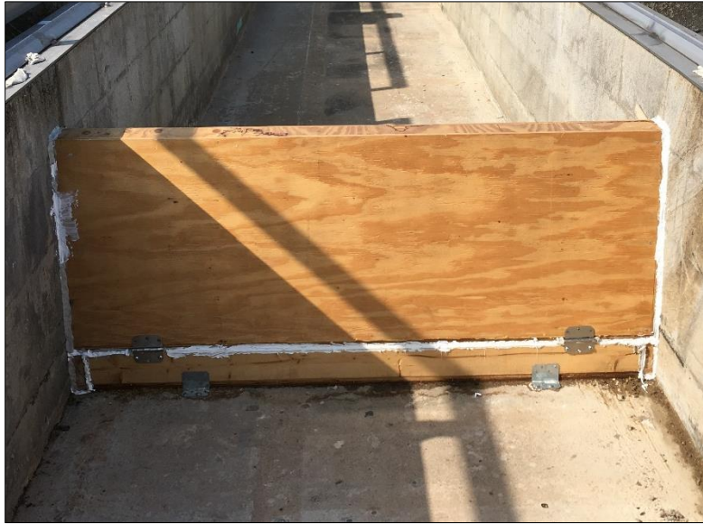
Figure 5.3. Weir Barrier.
