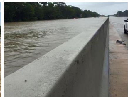
(b) The flooded westbound lanes of Interstate 12 with a concrete barrier damming up the flow of water (Louisiana) (3).
