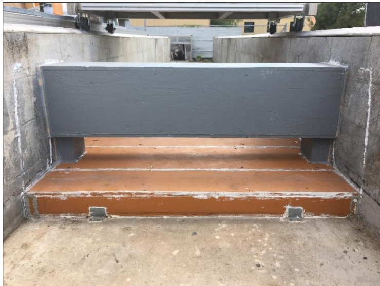
Figure 5.5. Post-and-Beam Barrier.
