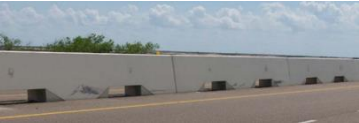
Figure 2.17. TxDOT SSCB (Wildlife Crossing).
