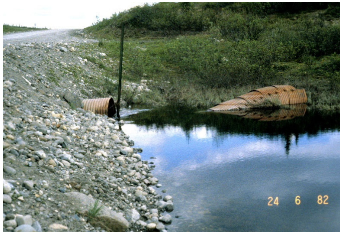
Figure 7-12 Settlement of inlet due to advection
