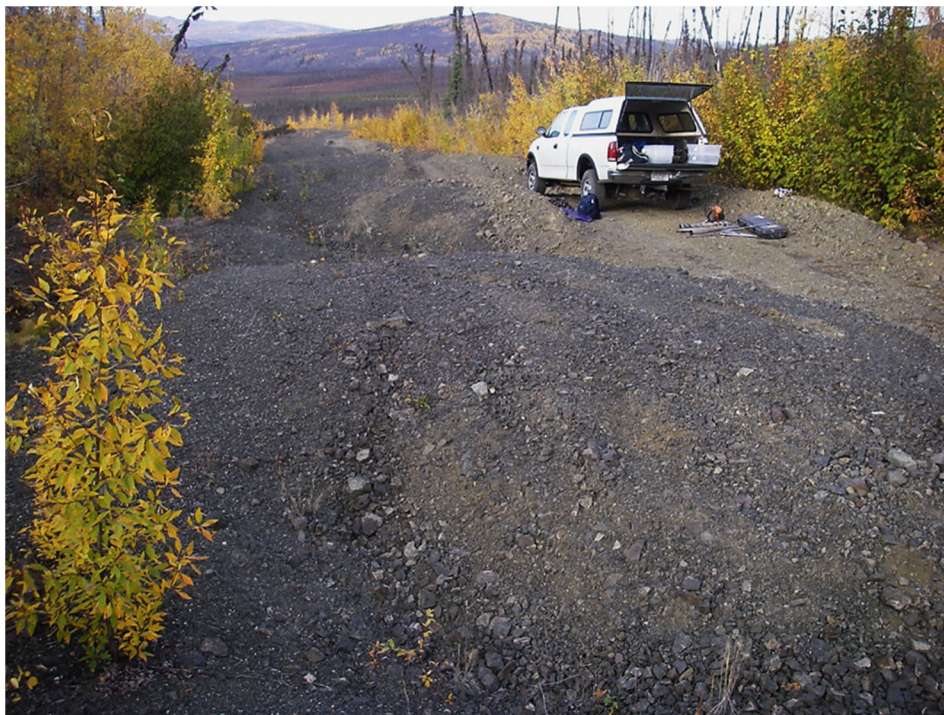
Figure 2-9 Thermokarst mounds (baydzherakhs) developed due to ice-wedge degradation under the abandoned part of the Dalton Highway, interior Alaska.
