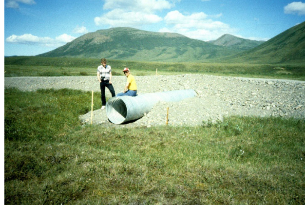
Figure 7-11 Culvert with extended outlet
