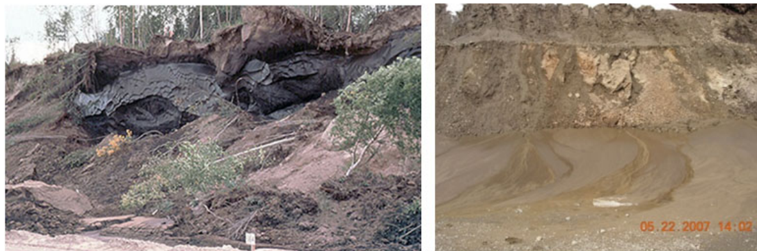
Figure 6-2 Massive ice exposed in cut slope (left) and runoff from thawing ice-rich cut slope (right).
