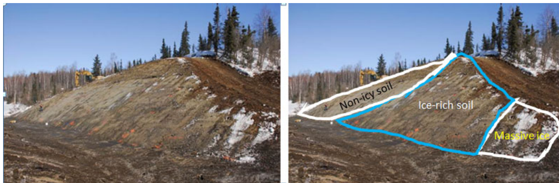
Figure 6-1 Three material types exposed in permafrost cut slope, prior to any thaw.
