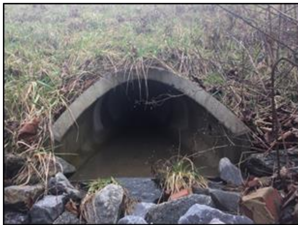
Figure 36. Photos. Bioretention basin test site at SR 113 and Racoon Creek, Bartow County .
