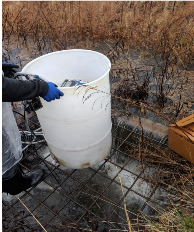
Figure 32. Photo. Overtopping of stormwater at the BMP outlet drainage control structure.
