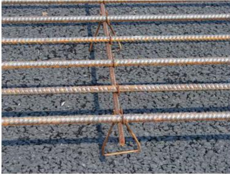
Figure 1. Photo. Longitudinal bars in CRCP. (Advanced Concrete Pavement Technology 2012)
