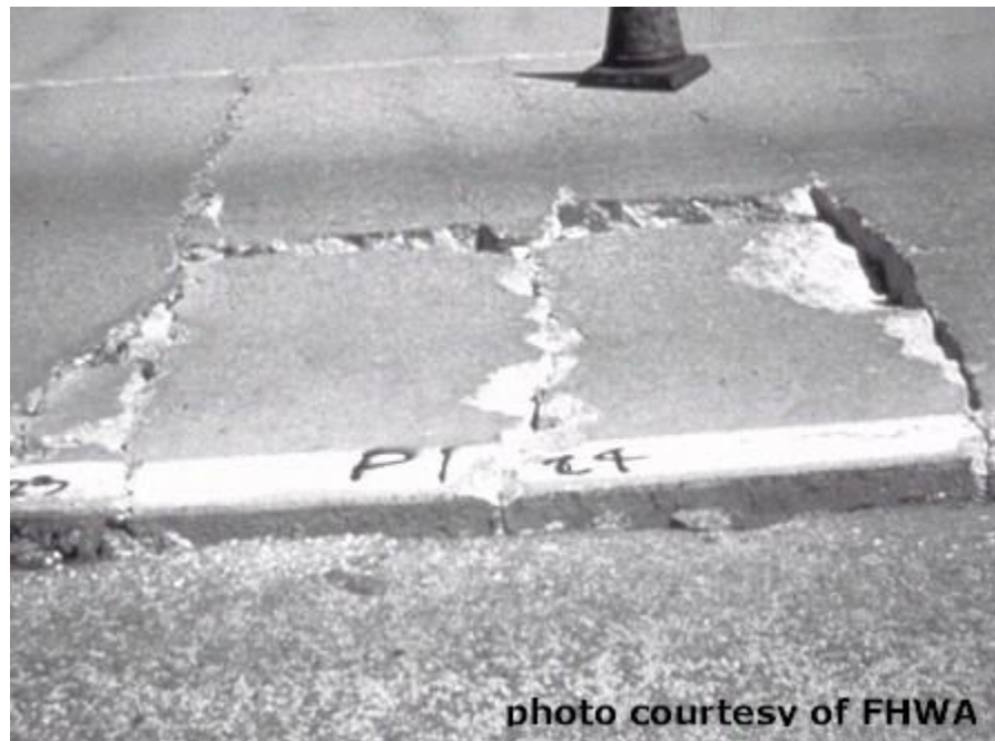
Figure 7. Photo. Example of punchout. (Pavement Interactive n.d.)
