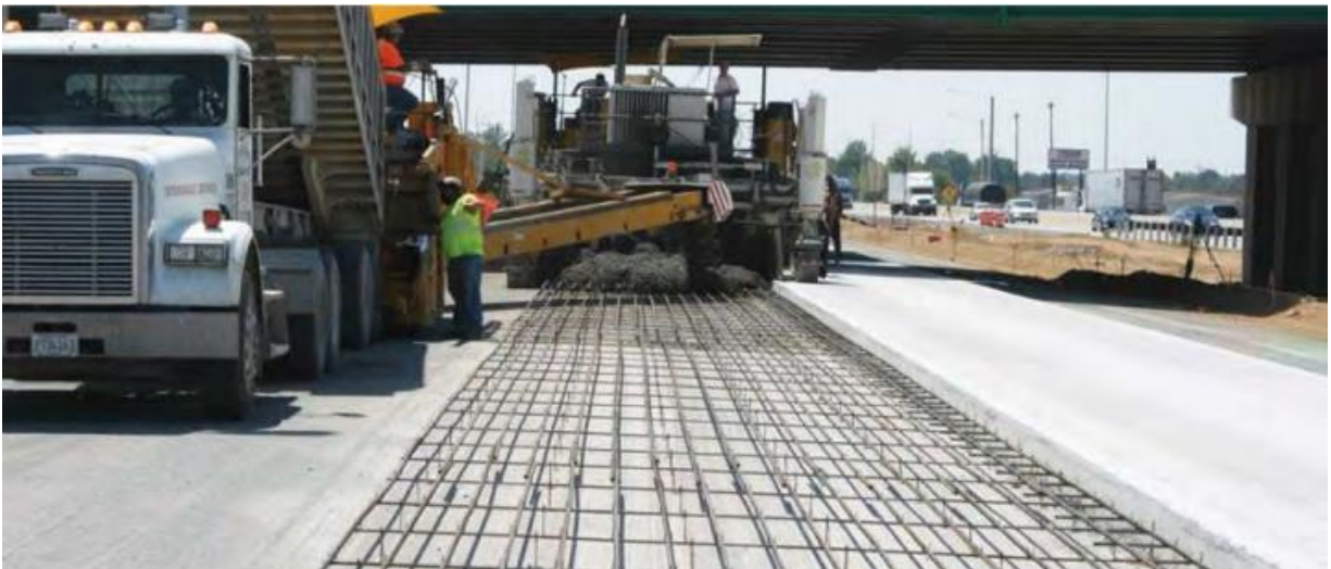
Figure 2. Photo. CRCP in construction. (Federal Highway Administration 2016)
