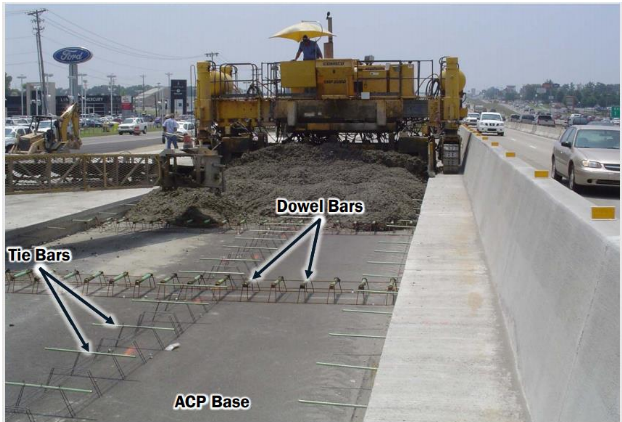
Figure 6. Photo. JPCP in construction. (Chen and Texas Department of Transportation 2013)
