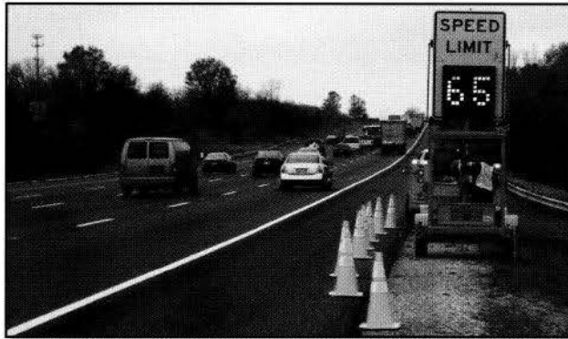
VSL trailer displays safe speed based on road work and traffic conditions
