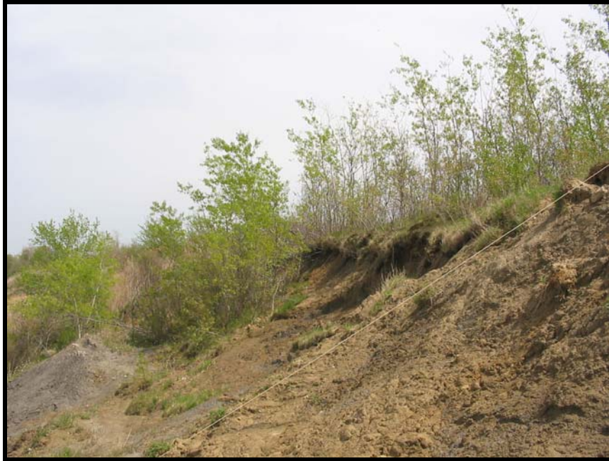
Figure 3.2 Slope with high potential to affect the roadway
