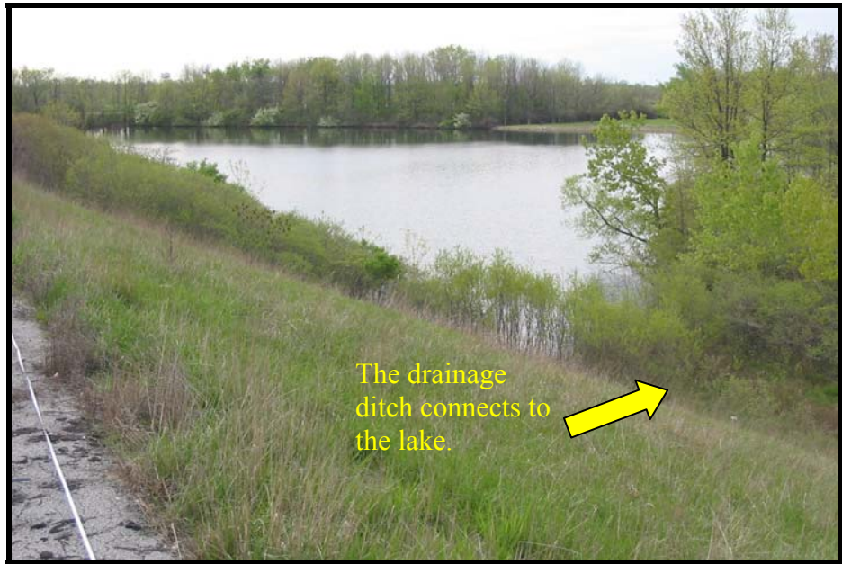
Figure 4.9 Lake at the toe of embankment
