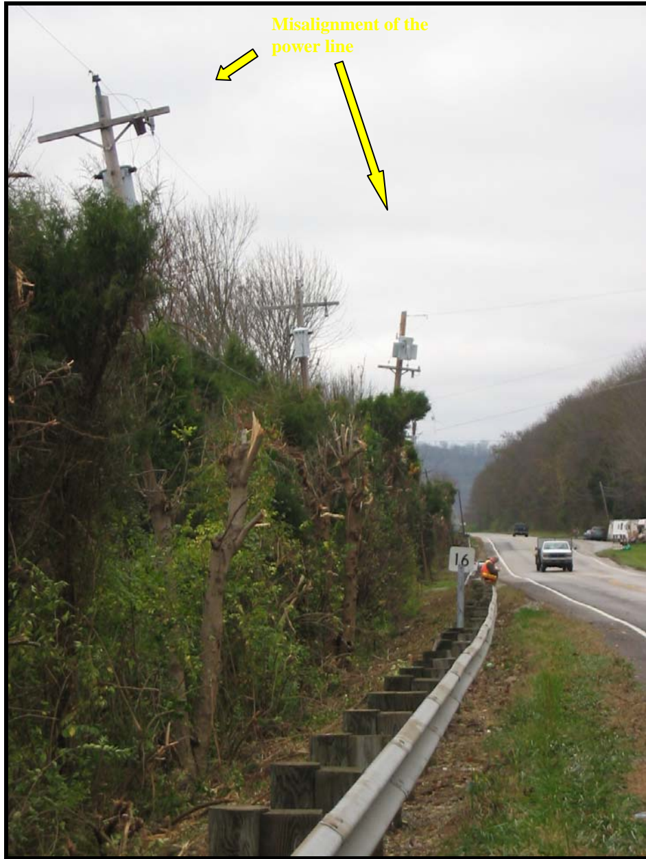
Figure 2.2 Misalignment of power line
