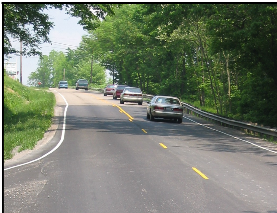
Figure 3.18 A restricted sight distance due to vertical curve
