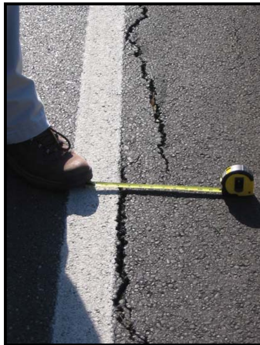
Figure 3.8 Displacement less than 1", receiving a risk score of 9 points
