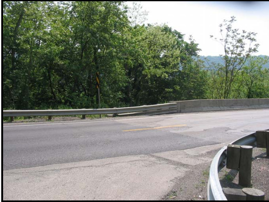
Figure 4.2 Southbound lane direction
