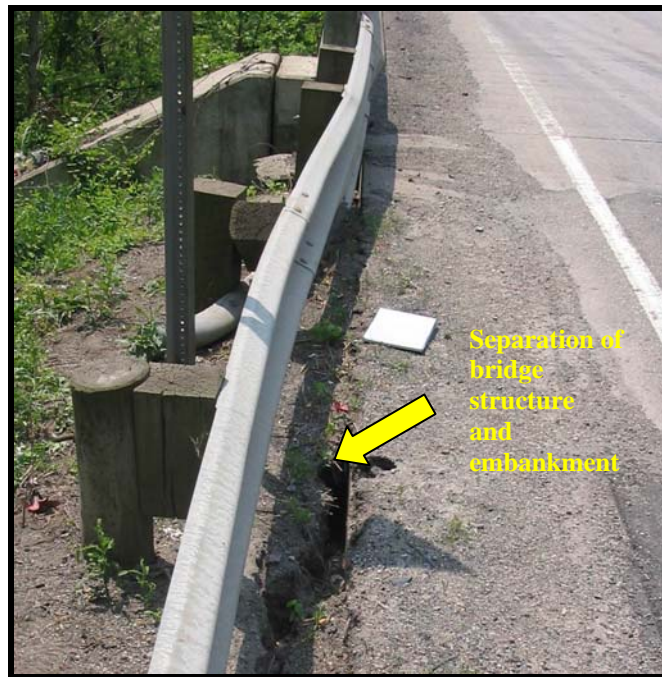
Figure 2.4 Separation of slope and bridge structure
