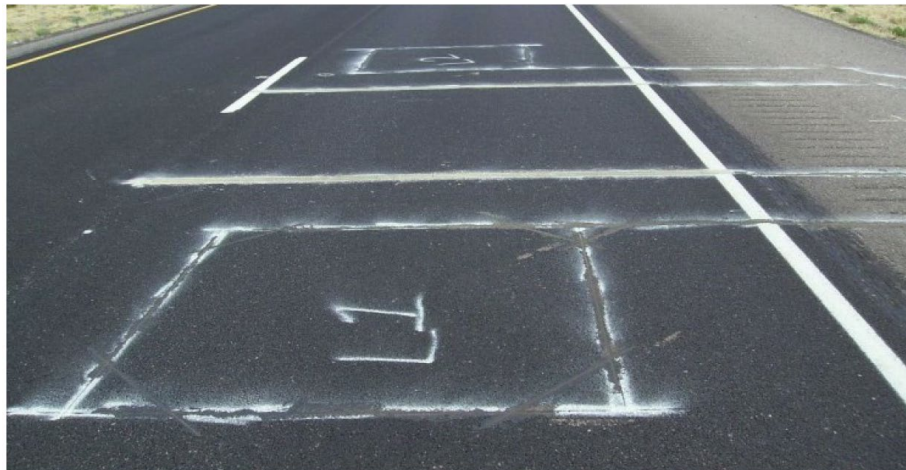
(b) Piezoelectric Weight Sensors (Type II)
