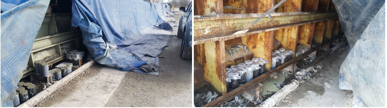
Figure 3-12. Concrete specimens stored under the tarps during curing the girders
