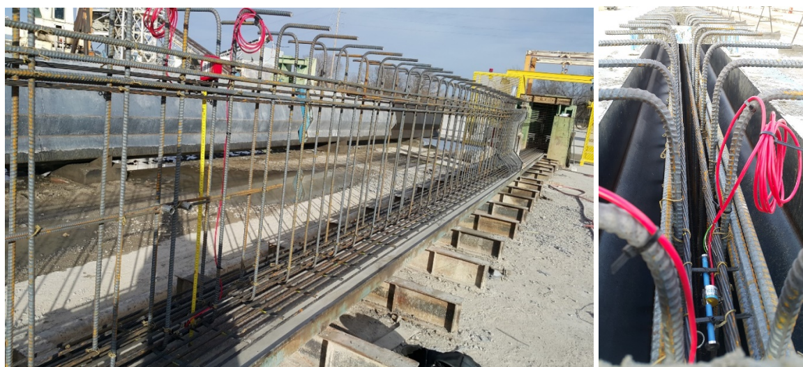
Figure 3-13. Strain gages attached to the prestressing strands
