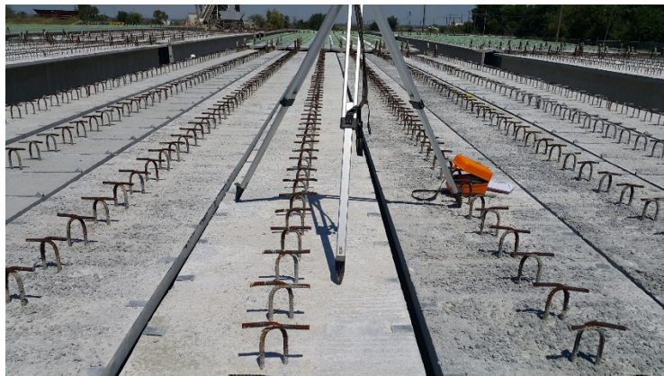
Figure 3-6. Automatic level positioned on top flanges surface to measure camber
