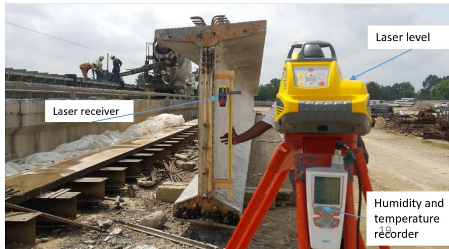
Figure 3-10. Rotary laser level and receiver rod used to measure camber
