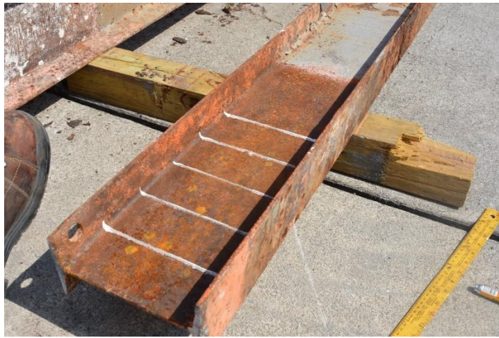
Figure 14. Specimen 1-S8-L Stripped of Paint
