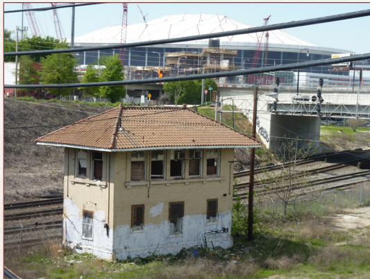
Atlanta Terminal Station interlocking tower (Fulton County)
