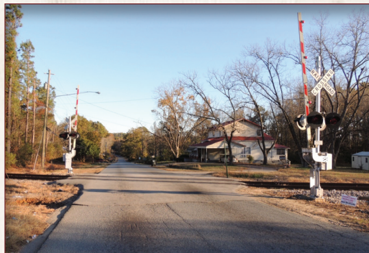
Typical grade crossing signals with gates, Cuthbert (Randolph County)
