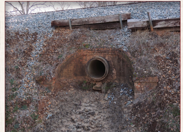
Brick and concrete culvert, Forsyth vicinity (Monroe County)
