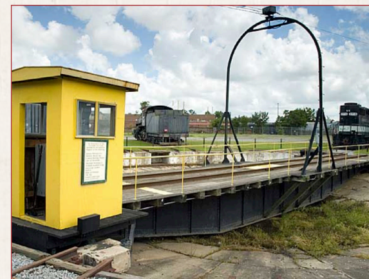
Turntable at Central of Georgia roundhouse in Savannah (Chatham County)
