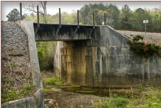
Concrete abutments for bridge over Dry Creek, Oakman vicinity (Gordon County)
