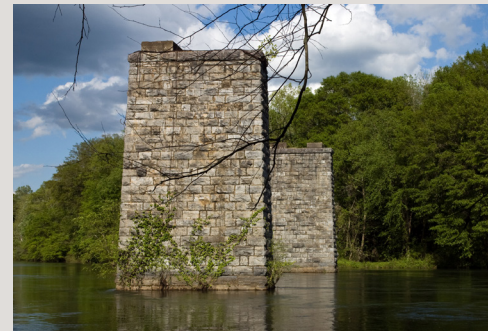
Etowah River bridge, Bartow County
