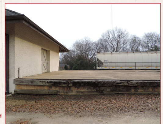
Concrete freight platform at Arlington Depot (Calhoun County)
