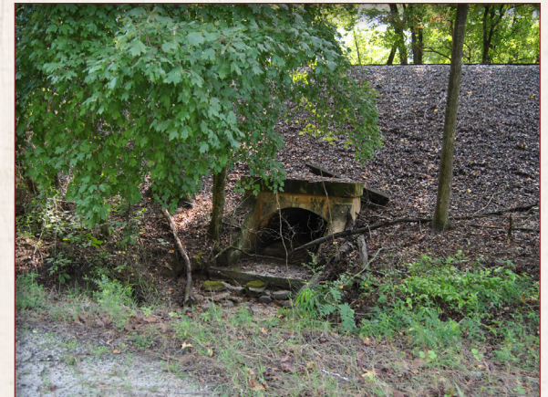
Concrete culvert near Barin Quarry in Columbus vicinity (Muscogee County)
