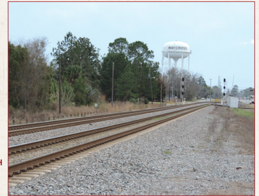
Double-tracked main line with concrete ties, Waycross/Hebardville (Ware County)
