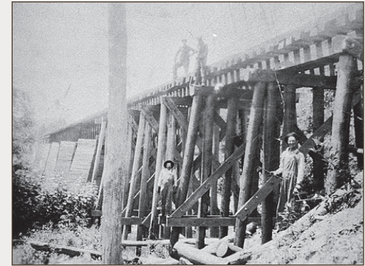
Trestle maintenance, Hall County, ca. 1926 (Vanishing Georgia)
