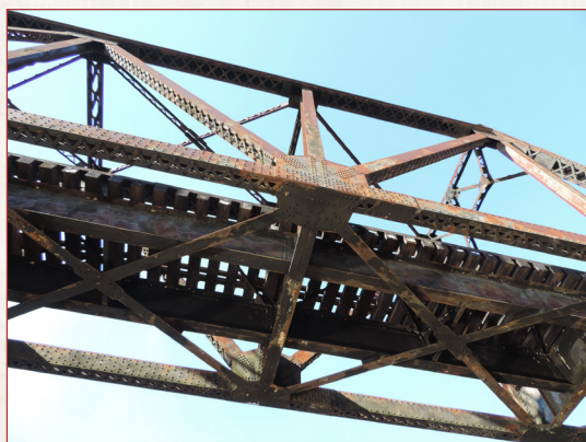
Through-truss bridge over Ocmulgee River, south of Lumber City (Telfair County)
