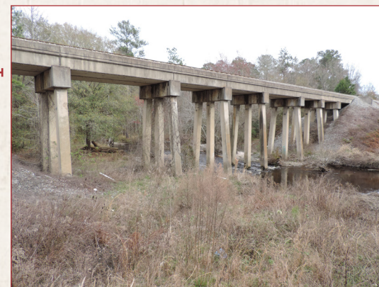
Concrete trestle bridge over Kettle Creek, near Jamestown (Ware County)
