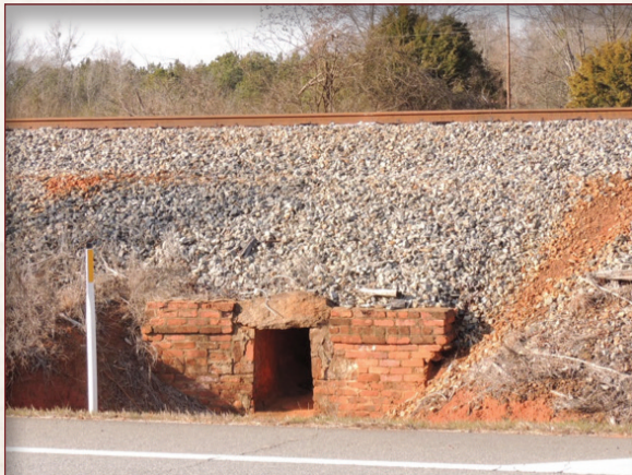
Brick culvert, The Rock vicinity (Upson County)
