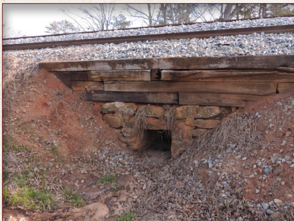
Stone and timber culvert, Griffin vicinity (Spalding County)
