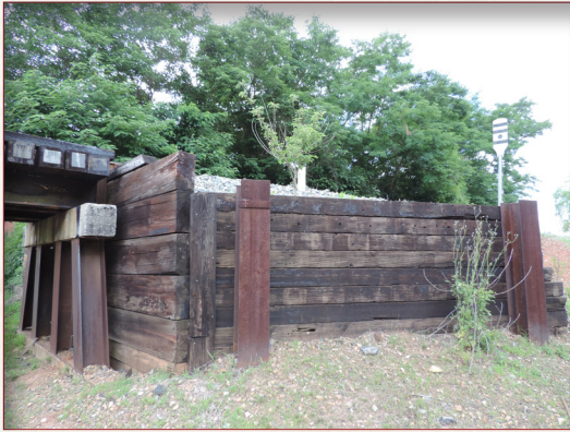
Timber abutment of trestle in Eatonton (Putnam County)
