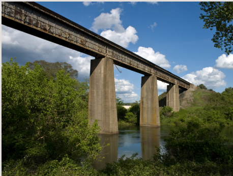
New Etowah River Bridge, Bartow County
