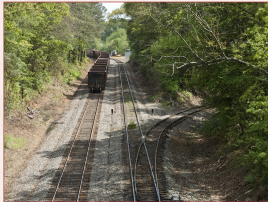
Spur track diverging to right, Cartersville vicinity (Bartow County)
