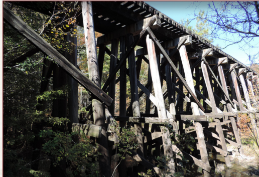
Bents of approach trestle to Altamaha River bridge (Jeff Davis County)
