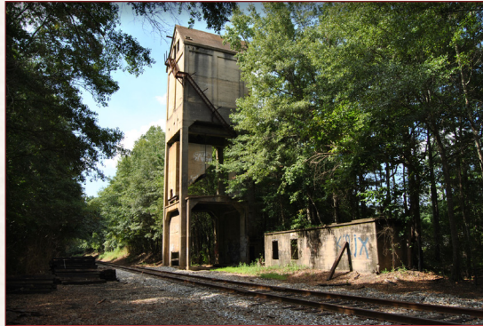
1926 Central of Georgia concrete coaling tower in Raymond (Coweta County)
