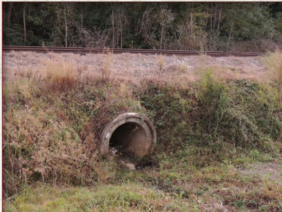
Concrete pipe culvert, Mt. Vernon vicinity (Montgomery County)
