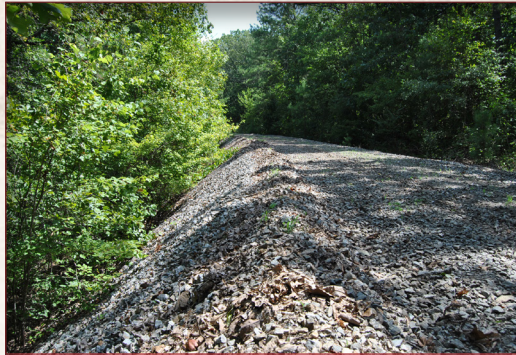
Remnant ballast of abandoned Central "R-line" near Pine Mountain (Harris County)
