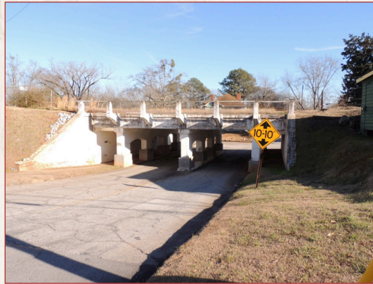
Viaduct of poured concrete at Palmetto (Fulton County)
