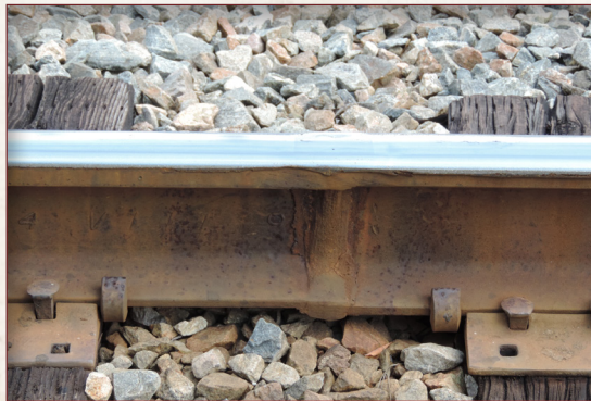
Welded rail on main line track at Dry Branch (Twiggs County)
