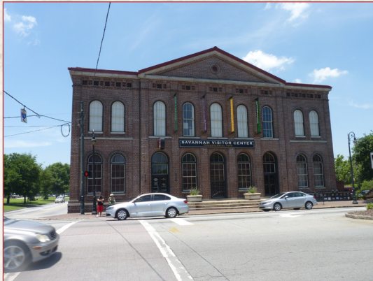
Head house of Central of Georgia passenger station in Savannah (Chatham County)
