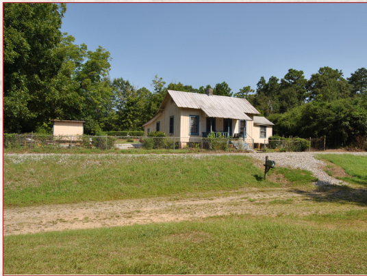
Former section house for railroad crew housing at Rehobeth (Harris County)
