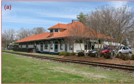
(a) An example of a combination depot at Lavonia. Freight room is on left. Depot agent's office and passenger waiting rooms are on right.
