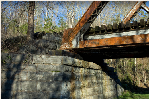
Masonry abutment of ashlar stone blocks, McCaysville vicinity (Fannin County)
