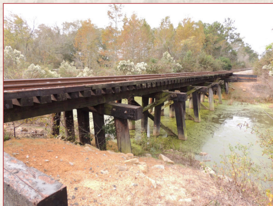
Timber trestle bridge in Wilcox County
