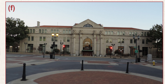
Macon Terminal Station
