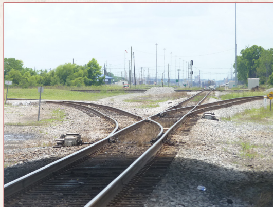
Wye junction into Rice Yard, Waycross (Ware County)
