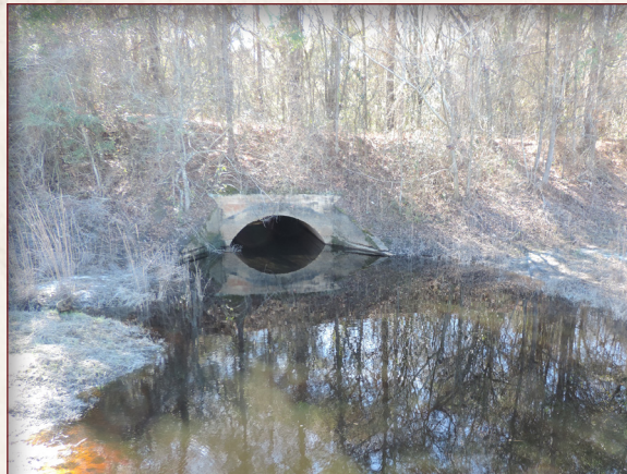
Concrete arched culvert in Willacoochee vicinity (Atkinson County)
