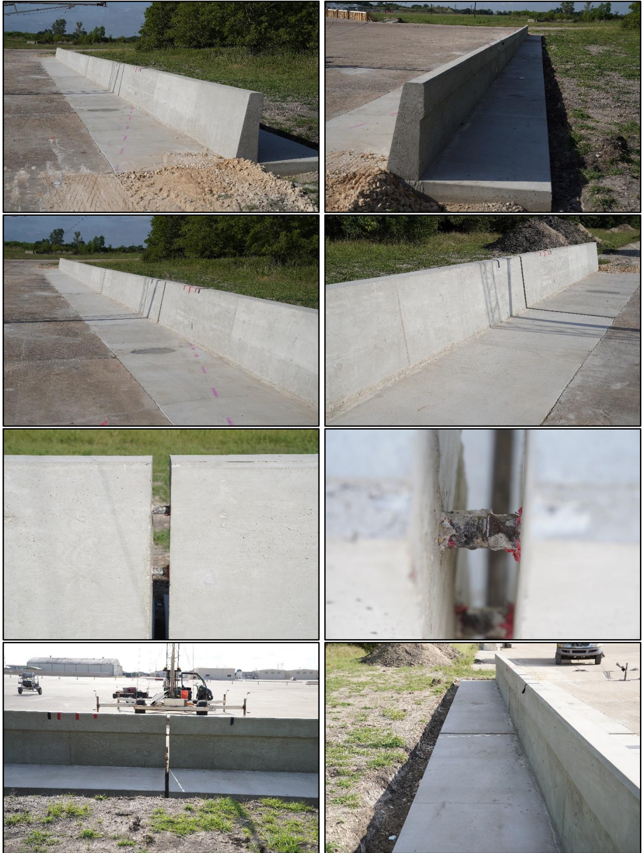
Figure 2.2. TxDOT Shallow Anchorage SSTR prior to Testing.
