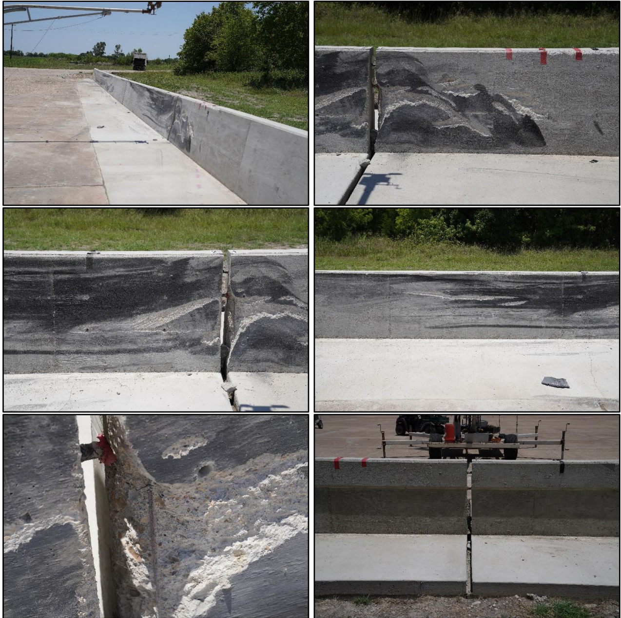
Figure 5.3. TxDOT Shallow Anchorage SSSTR after Test No. 469680-02-1.
